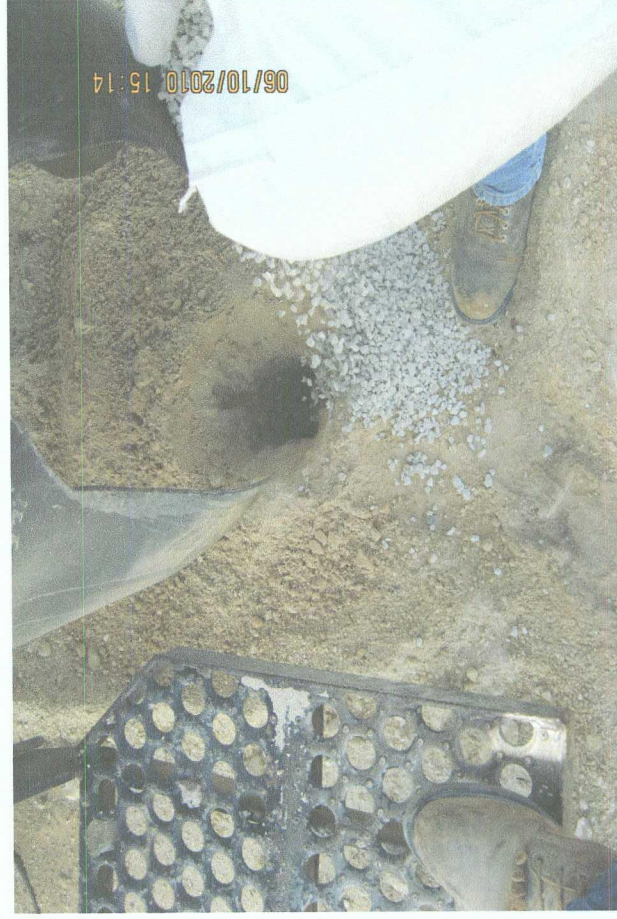
Soil bore # 1 plugged with bentonite
