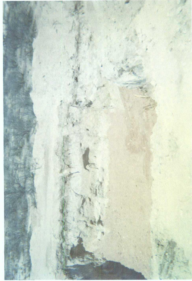
Clay liner installed
