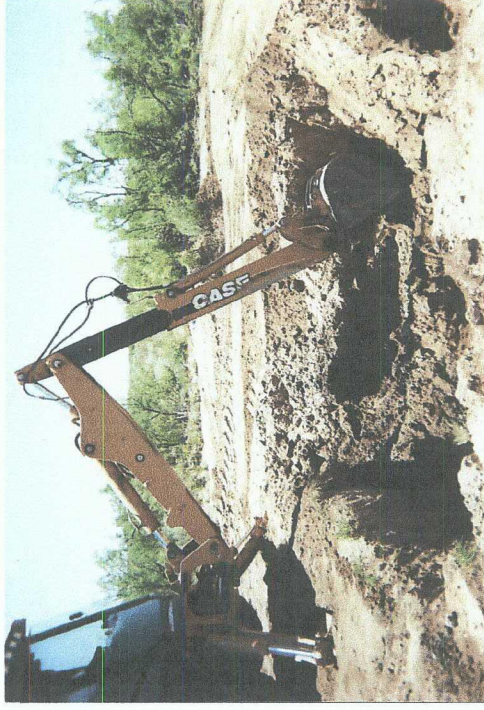
Delineation trench being excavated
