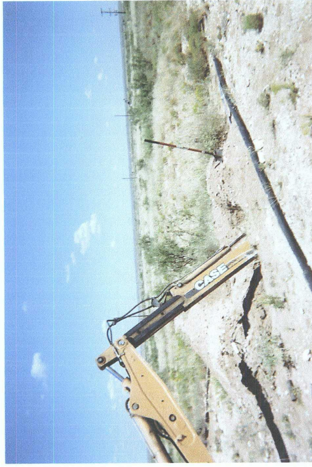
Delineation Trench being excavated
