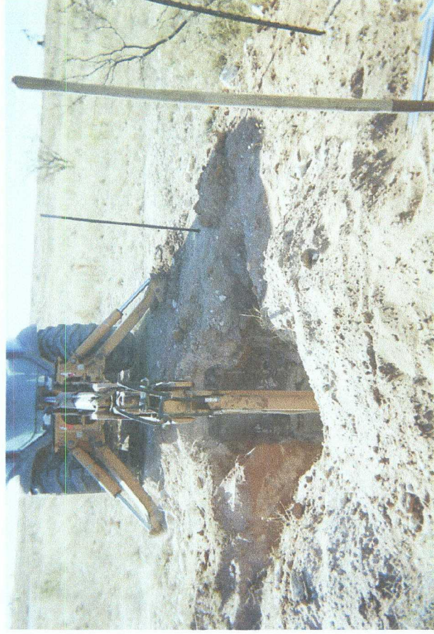
Delineation trench being excavated
