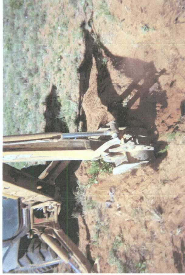
Delineation trench being excavated
