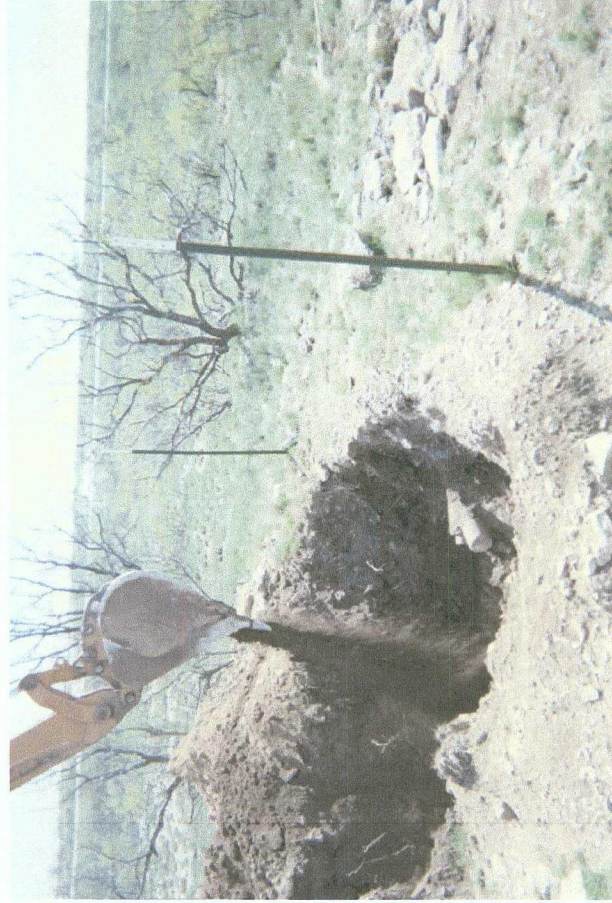
Backfilling excavation
