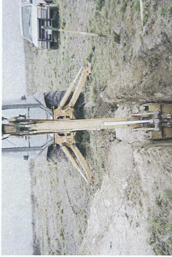
Delineation trench being excavated
