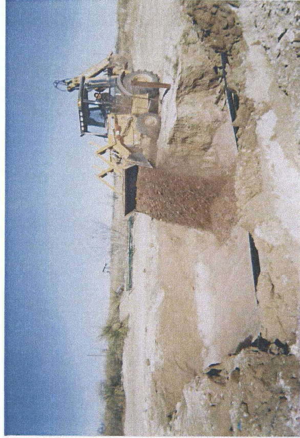
Installing clay liner
