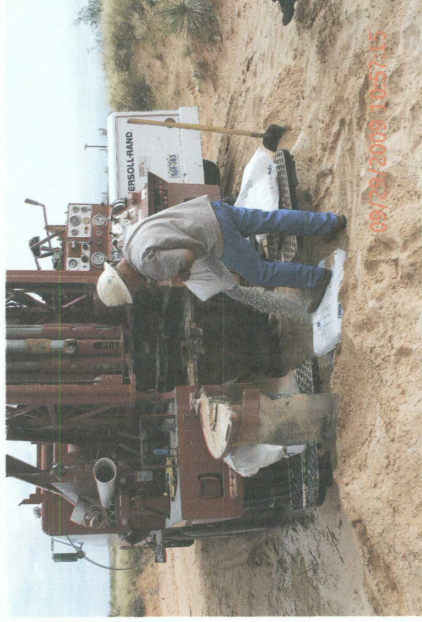
Plugging bore with bentonite
