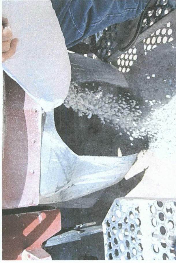
Plugging the bore hole with Bentonite
