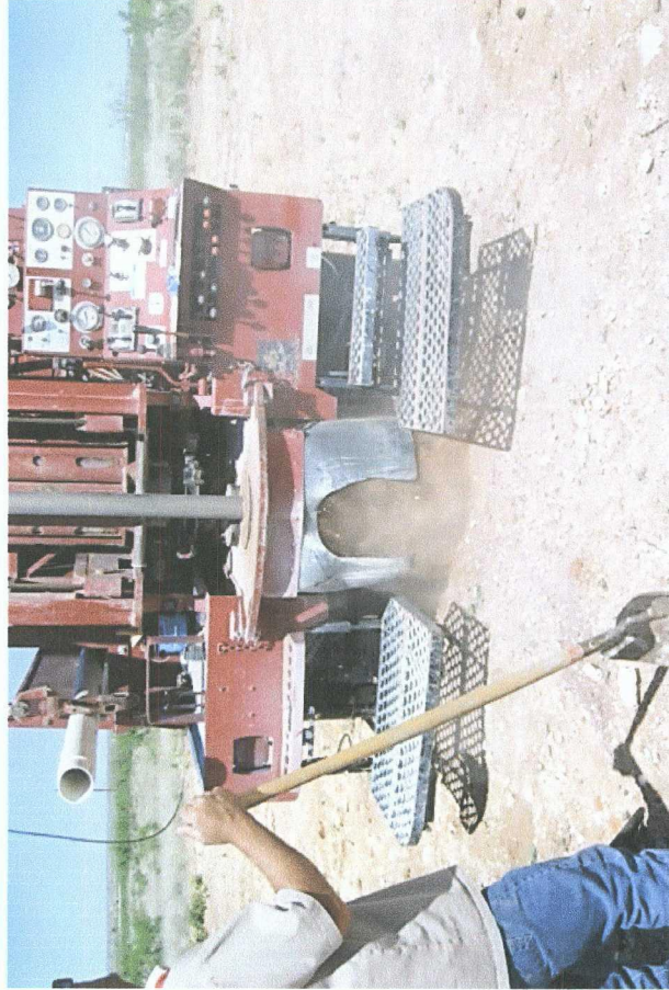
Drilling the bore hole
