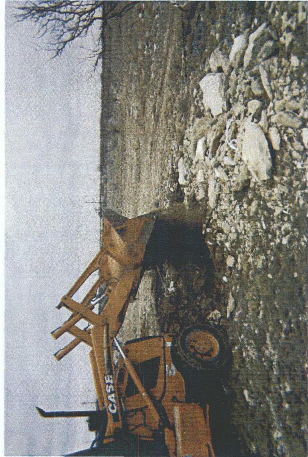
Backfilling excavation
