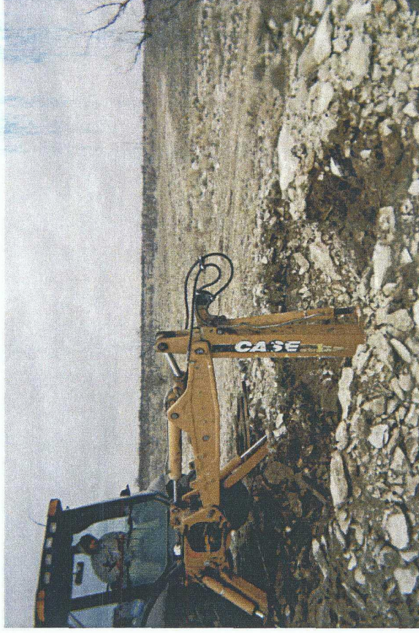
Delineation trench at former junction box
