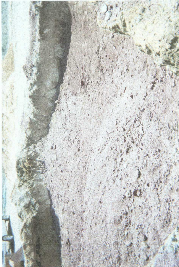
Clay layer installed
