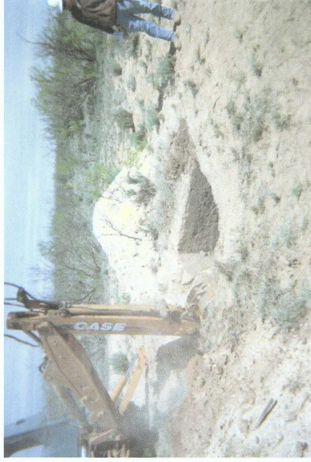
Delineation trench being excavated
