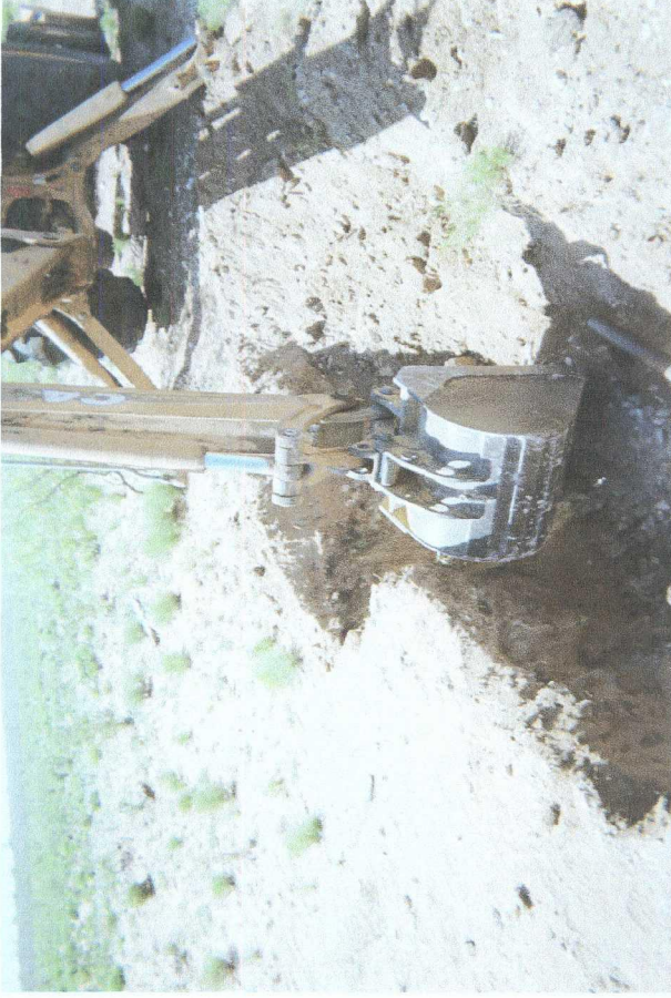
Delineation trench being excavated
