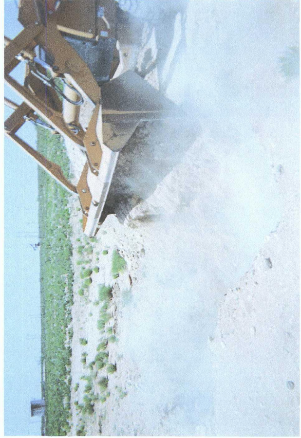
Backfilling excavation
