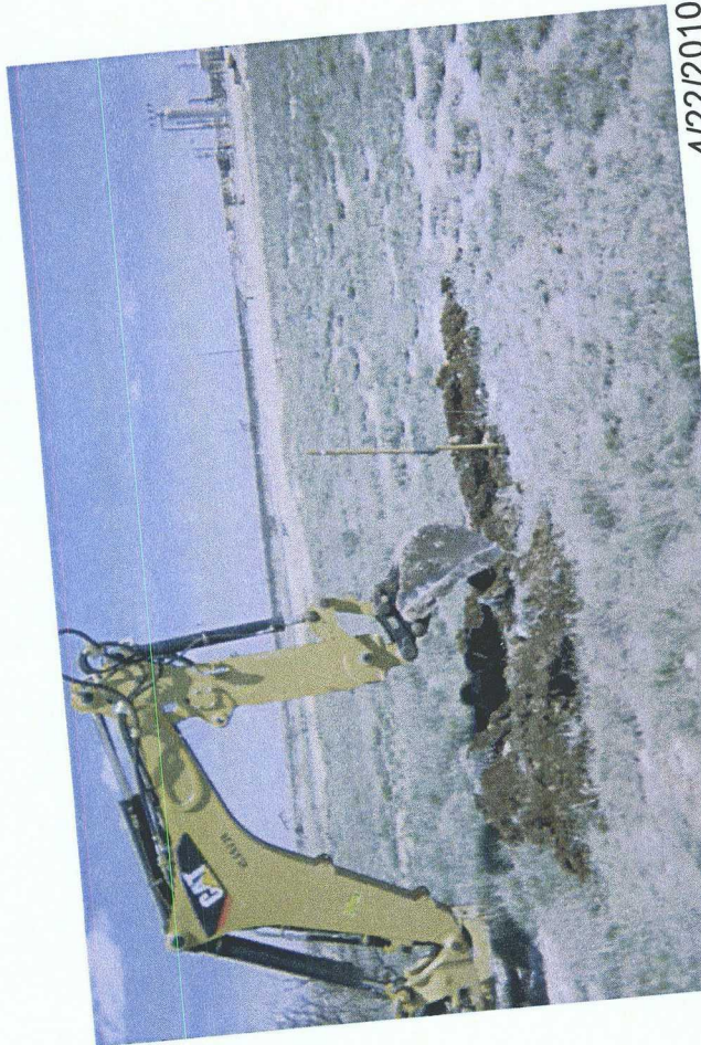
Delineation trench being excavated
