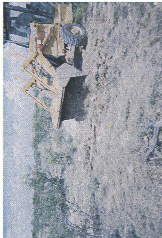
Backfilling excavation
