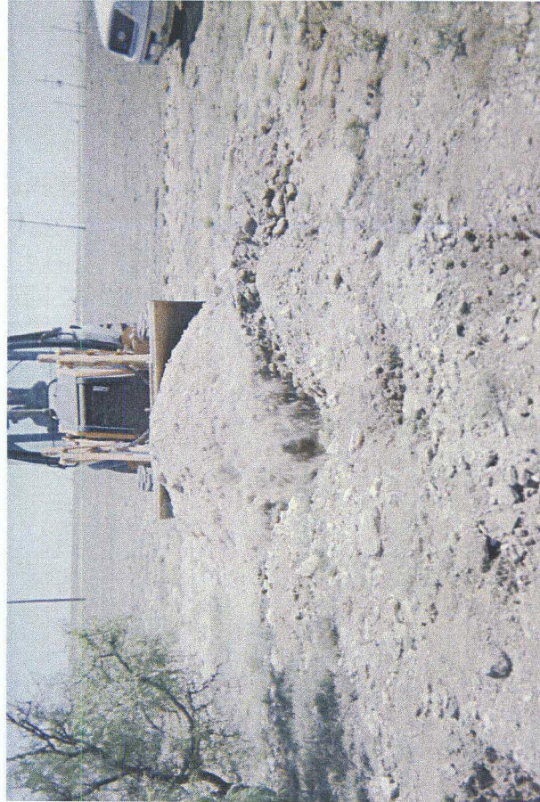
Backfilling excavation
