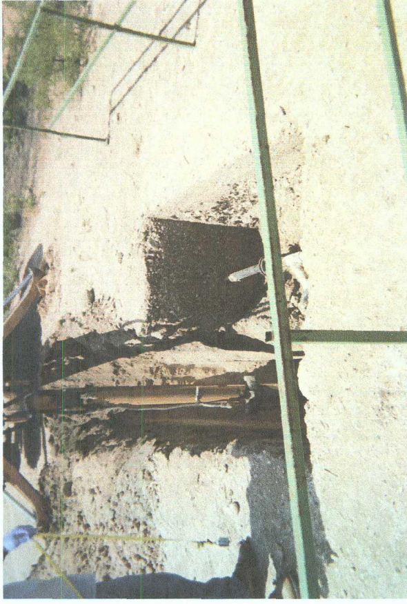
Delineation trench being excavated
