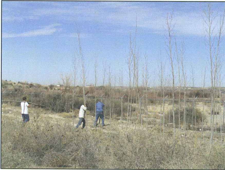
March 15, 2011: BioTech and NMSU personnel planting trees in pre-bored 7-foot holes. Groundwater was encountered between 4 and 5 feet below ground surface.
