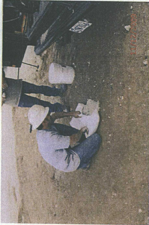
Plugging entire soil bore with bentonite
