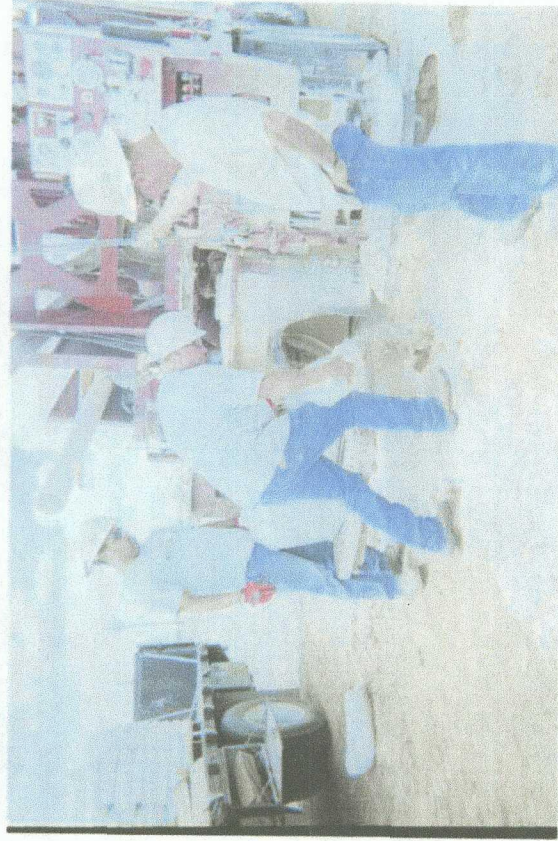
plugging SB #1 with bentonite
