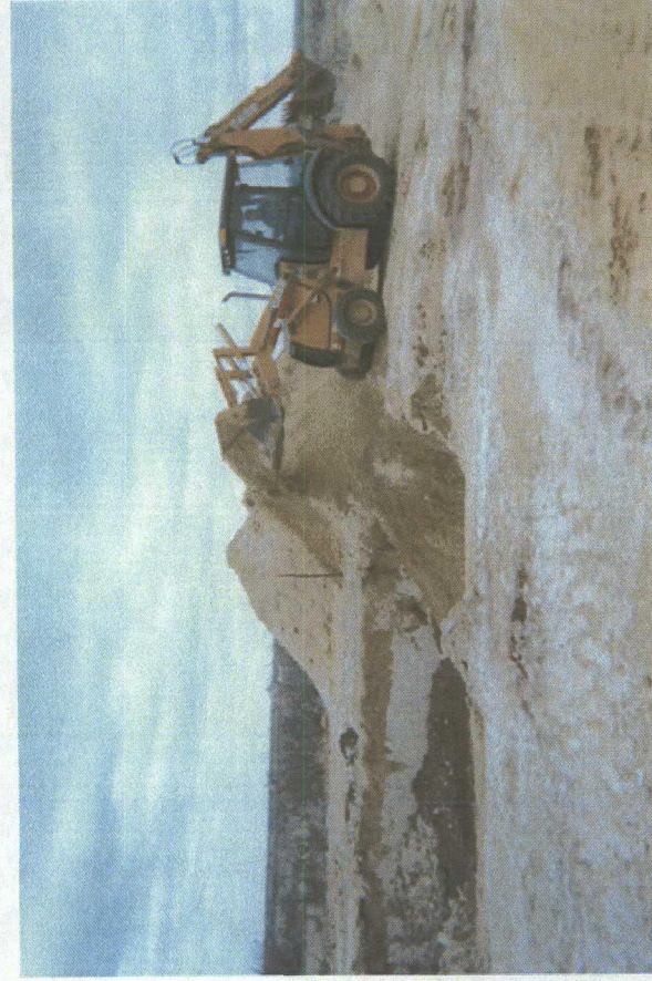
Backfilling excavation
