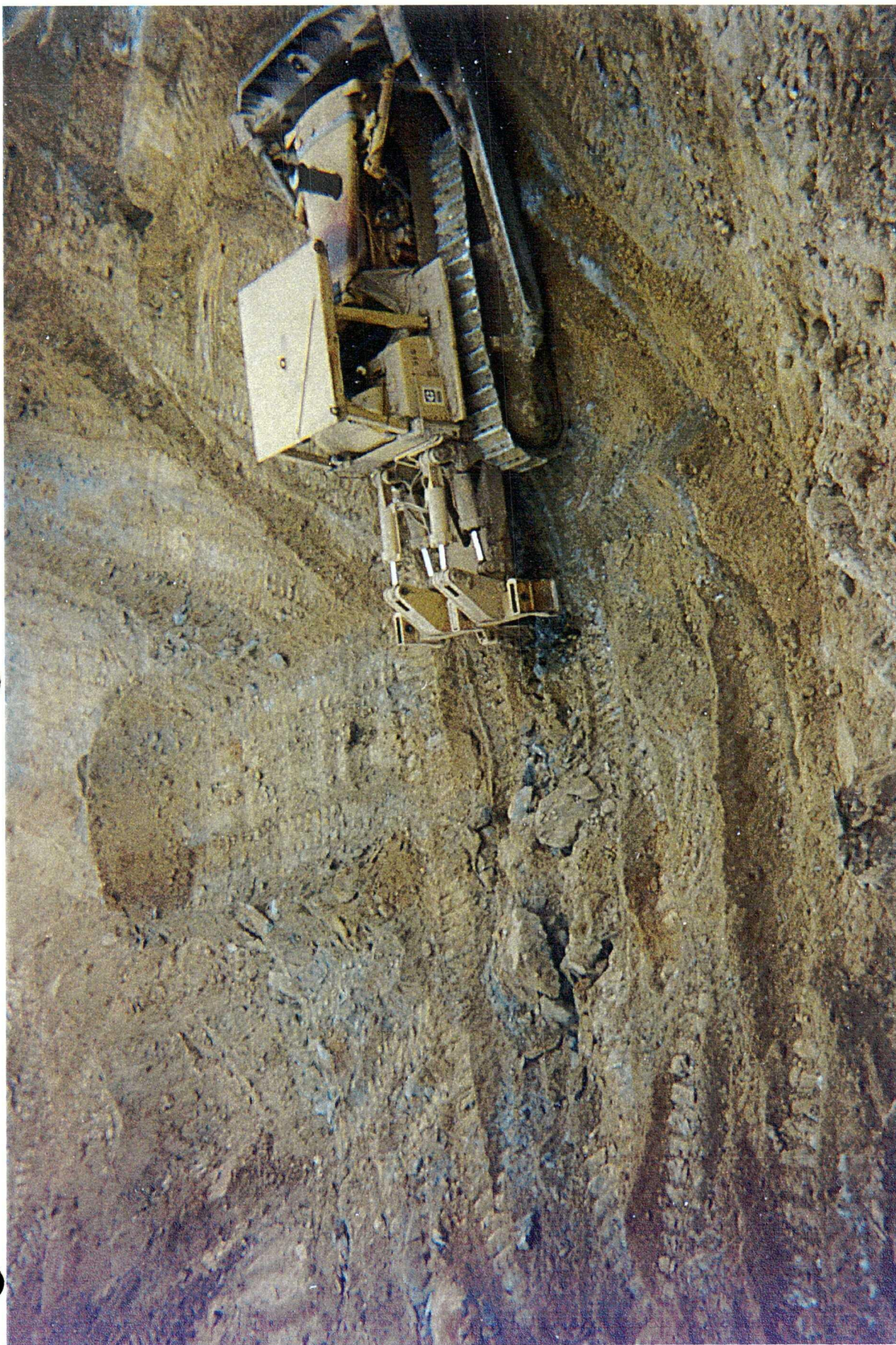
Hampton 4M, looking down into excavation Native soil beneath PNM's former pit
