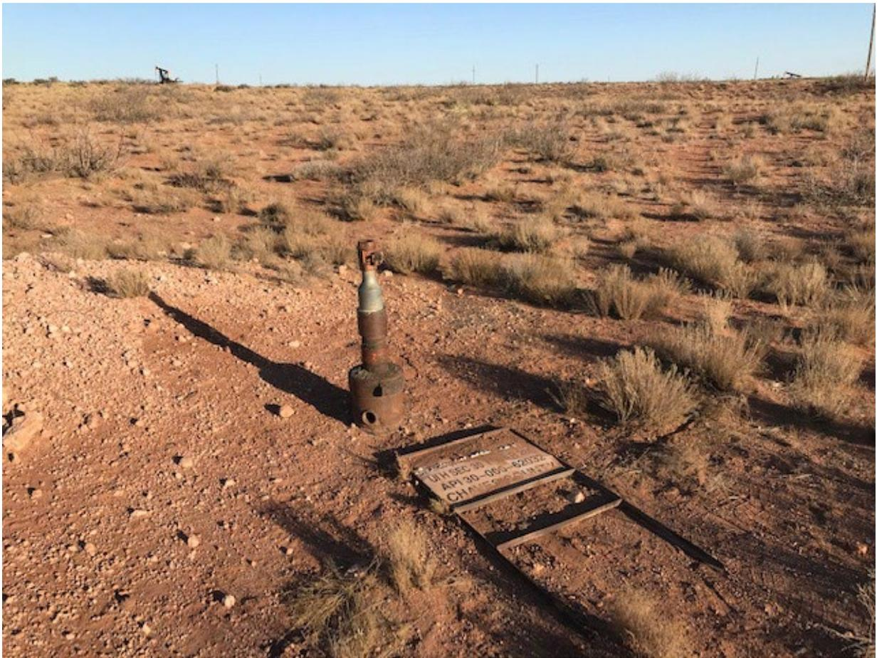
**Plains #29-4 (30-005-61904). No rods or valve on tubing (2 photos).**
