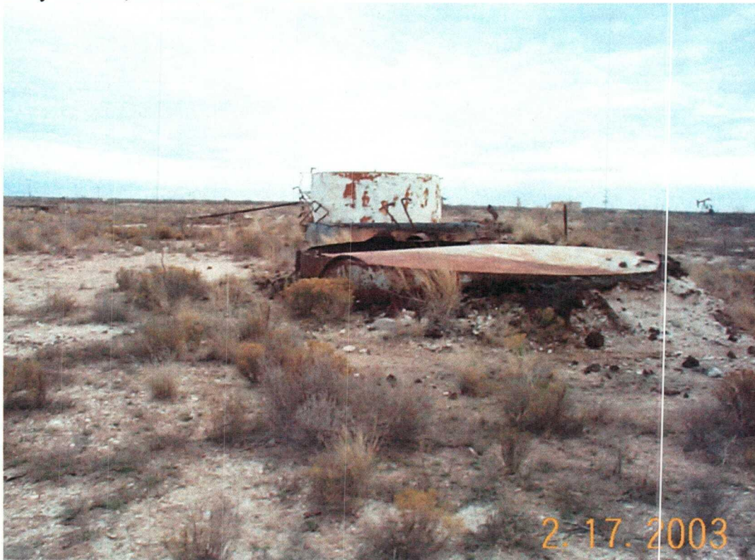
Photo 1: 2- Buried 250 bbl tanks containing paraffin and water, 1-insulated 250 bbl tank contents unknown. Looking East
