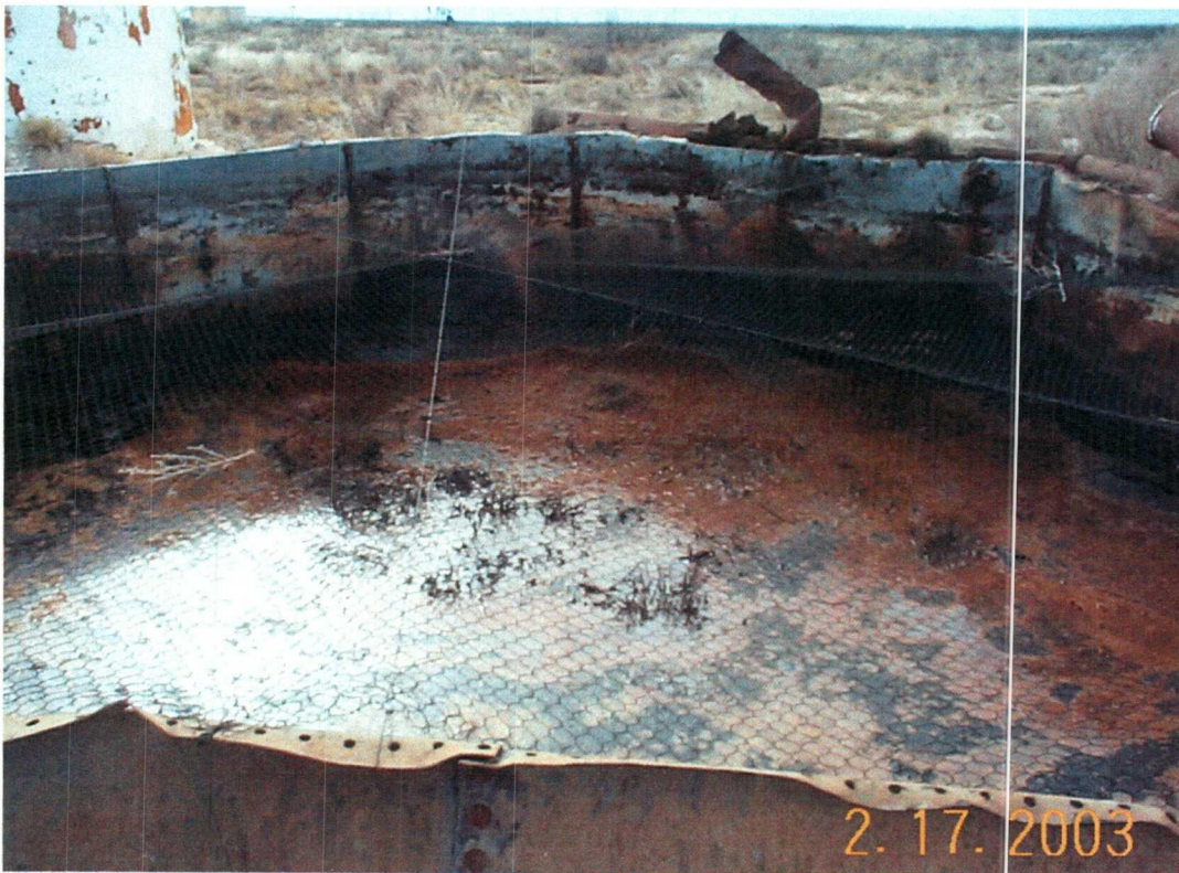
Photo 2. Close up of buried 250 bbl tank with net and fluid. Looking Southeast.
