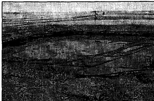
Poorly installed and maintained netting at this commercial oil field produced water disposal facility in Wyoming allows entry by migratory birds and other wildlife. To insure effectiveness, netting should exclude wildlife from ground as well as aerial entry.
