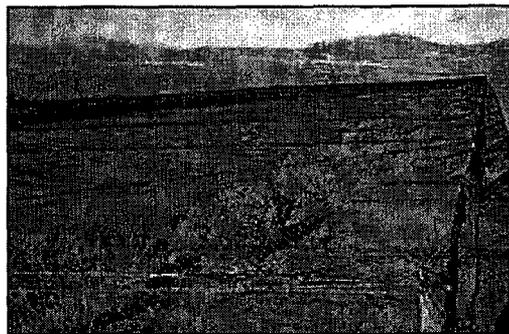
Properly installed net at commercial oil field produced water disposal facility in Wyoming. Net is supported by steel frame and high-tensile strength cable to prevent sagging. Sides are also netted to prevent ground entry by birds and other wildlife. Netting to exclude migratory birds should also extend down the sides of the supporting frame to prevent ground entry by birds and other wildlife
