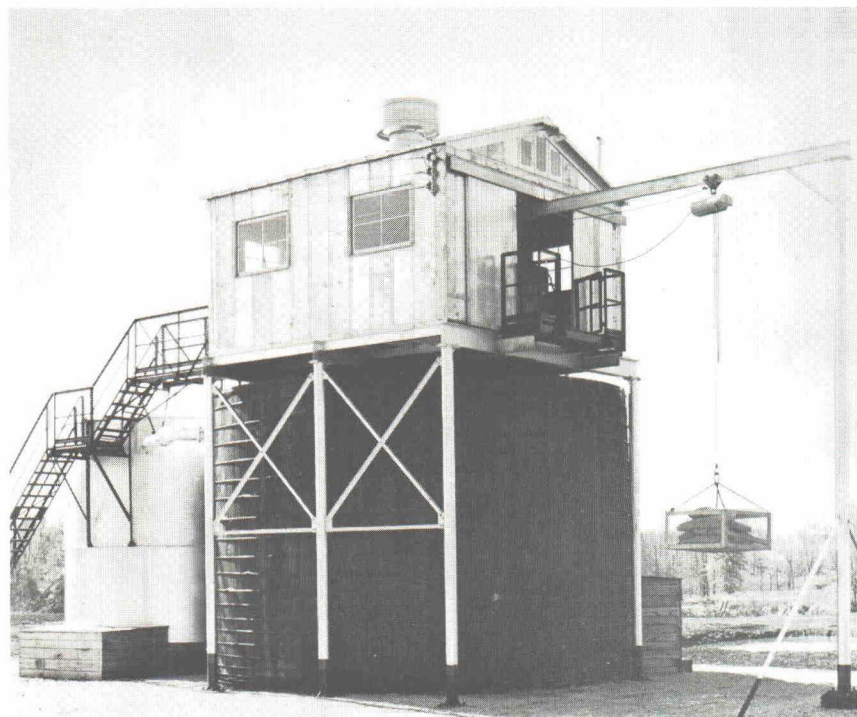
24' x 16' "National" Stabilization and Clarification System designed in a Redwood Tank for extremely corrosive water. Two dry chemicals are automatically fed within the externally supported process control and chemical storage building. Purified water surge tank is located beside the processing system. This entire system was designed and constructed by National Tank Company.
