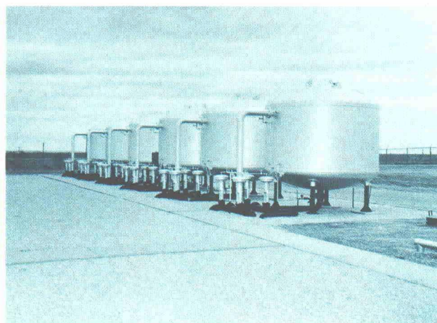
6 — 10' x 5' 40 psi filters with anodes and singly operated diaphragm butterfly valves in an automated filter manifold.
