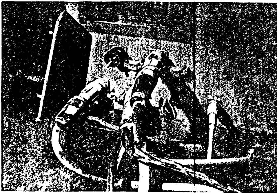
East end of the No. 2 portable load center with cables coming from nips.
