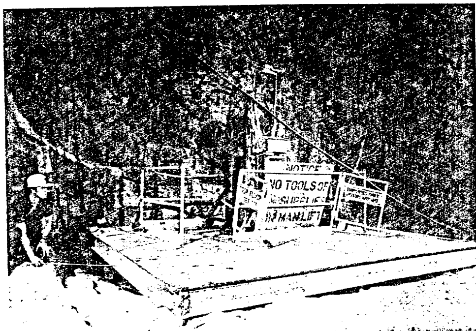
Top of manlift at 2 Main Entry East just west of 1 Main Entry South. Entire frame moved to the west 2 feet.
