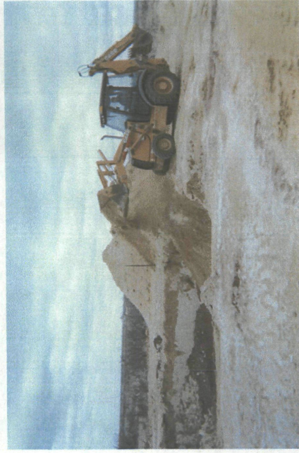
Backfilling excavation
