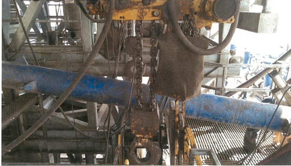
Figure 2: BOP Winch System
