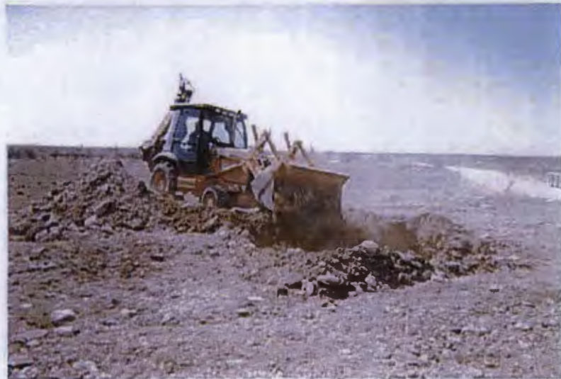
Backfilling excavation
