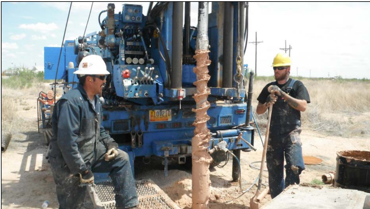
No. 2 – Wet, clayey soils from MW-07.
