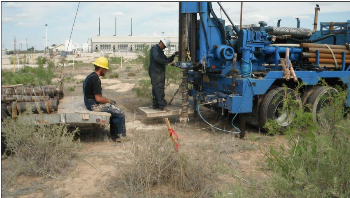
No. 3 – Commencing to drill at MW-11.
