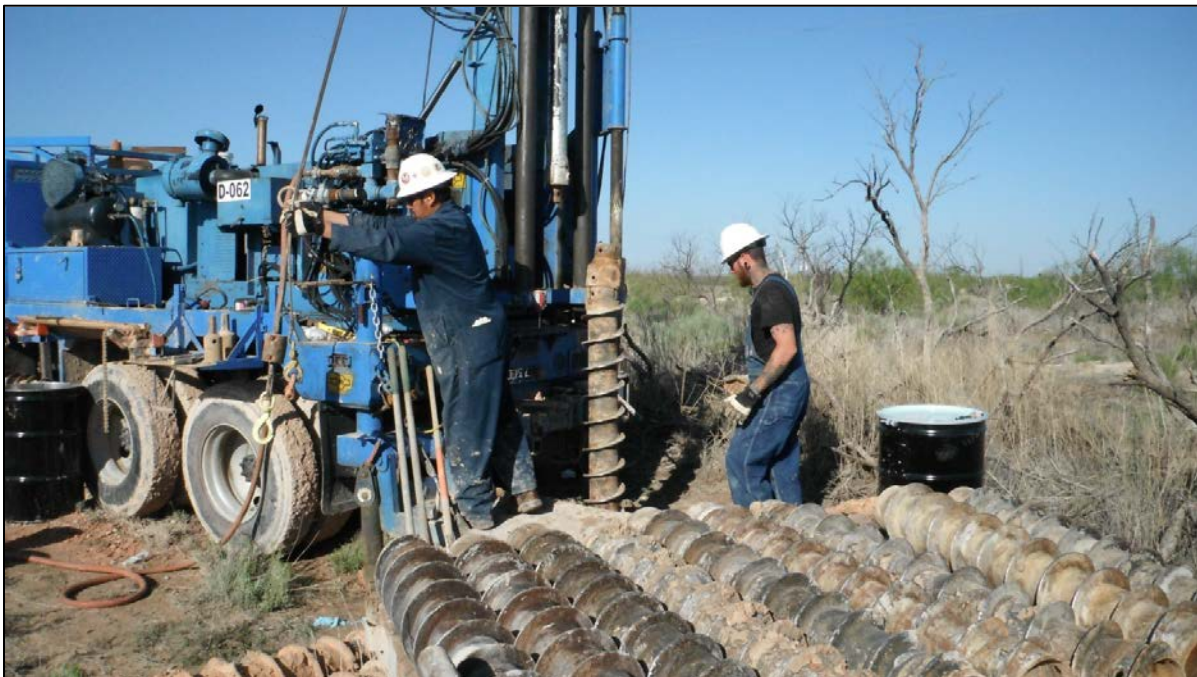
No. 10 – Preparing to over-ream MW-10 from a diameter of approximately 8-inches to a diameter of approximately 10 inches.
