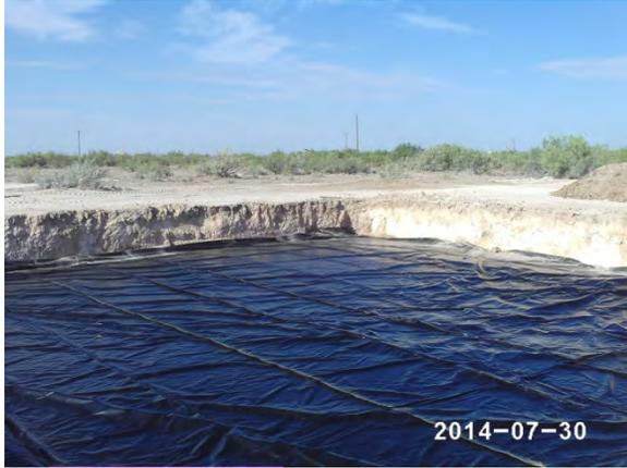
20-mil poly liner installed at 4.5 ft bgs,
