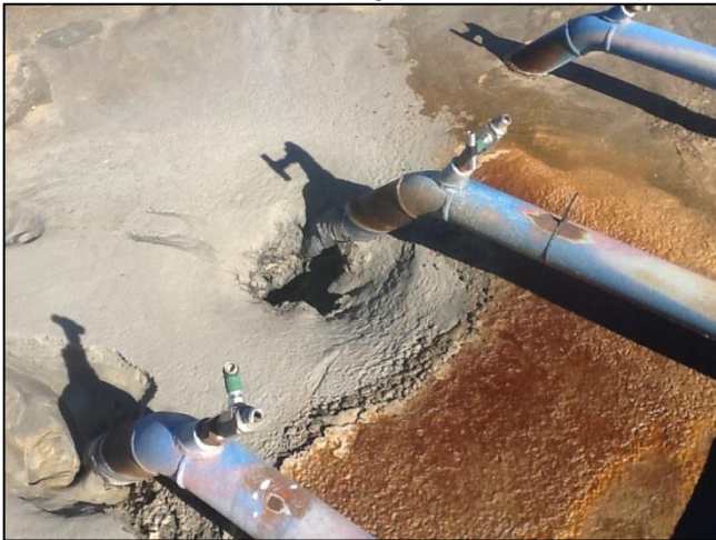
Saturated soil at leak location (Photo # 3)
