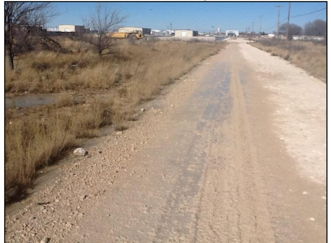
Ponding and saturated soil on lease road looking north (Photo # 12)
