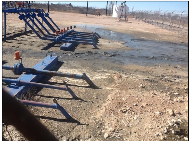
Ponded and saturated soil at manifold facing west (Photo # 4)
