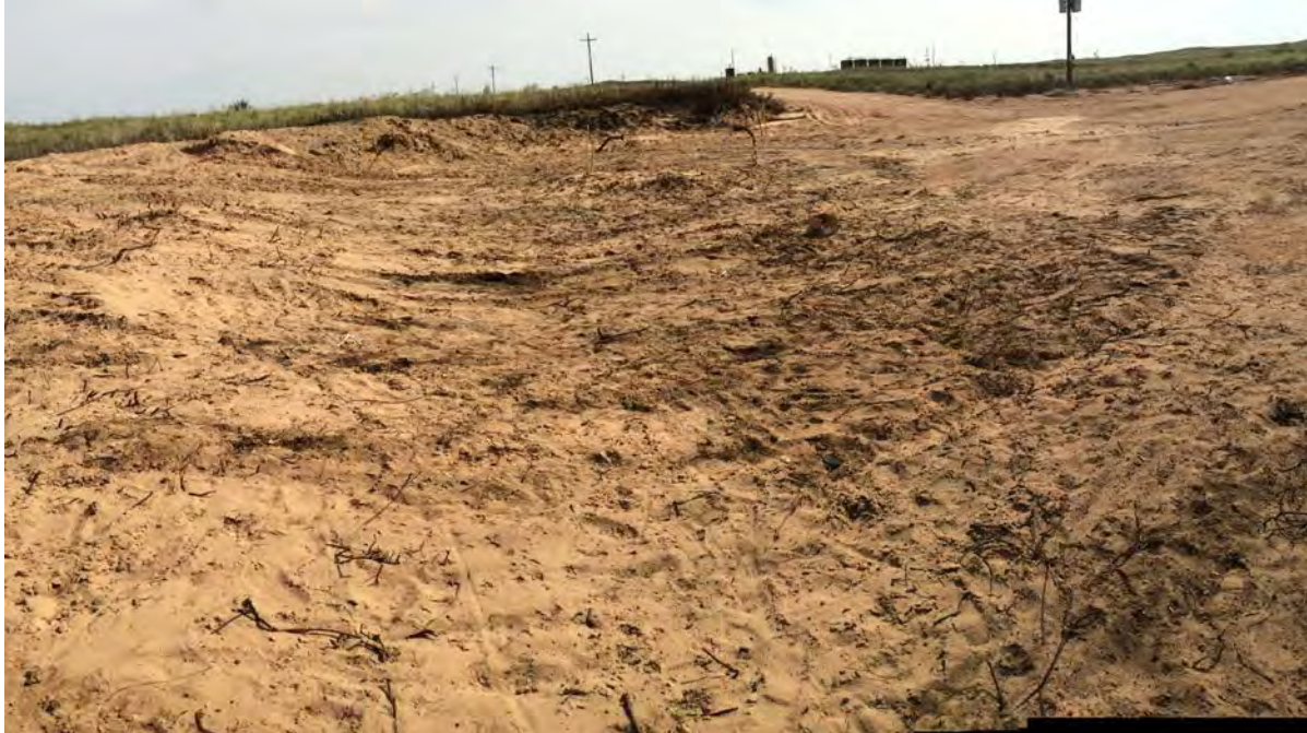
Figure 3 – View to the south from the same location as Figure 1. The initial response removed as much liquid crude as possible with a backhoe, creating a stockpile of impaired material near the heater treater. The area of impact (ash and residual oil) was then dragged by the end-loader of the backhoe to cover the crude to reduce the potential of exposure to cattle.
