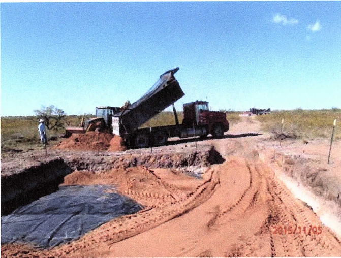
Padding above the liner with imported blow sand, facing northwest 11/5/2015
