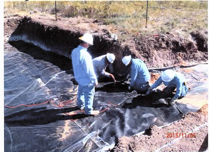
Seaming the liner, facing east 11/5/2015
