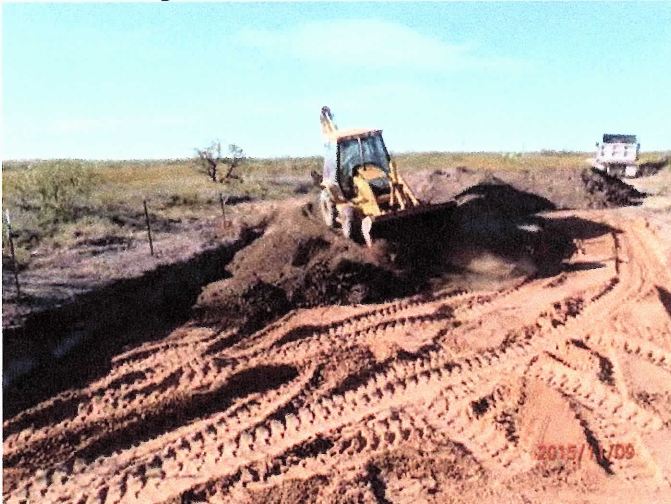
Backfilling with imported top soil, facing northwest 11/9/2015
