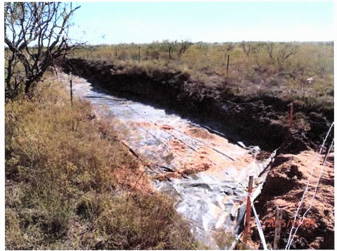
20-mil, reinforced liner installed in the south half of the site, facing south 11/9/2015
