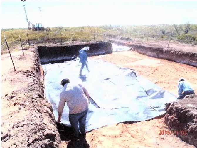
Installing a 20-mil, reinforced liner above a 6 inch pad of blow sand, facing south 11/5/2015
