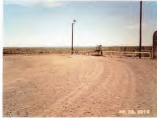
East Load Pad Driveway-Looking ESE
