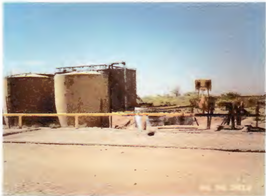
West Load Pad-Looking South
