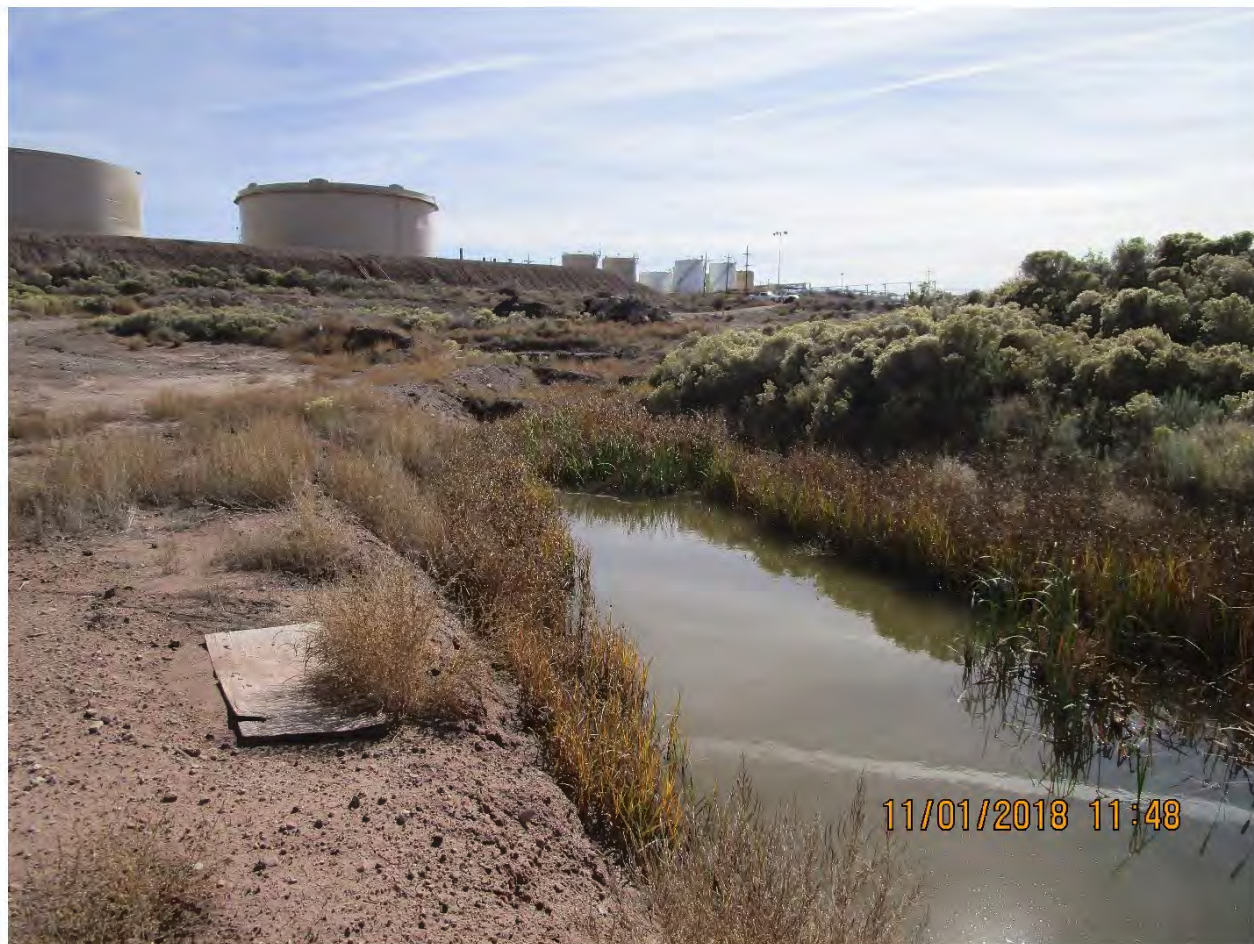
Photo of lowermost (northern) end of retention ditch. Oil stained vegetation shown around edges of ditch but no recoverable product on water.
