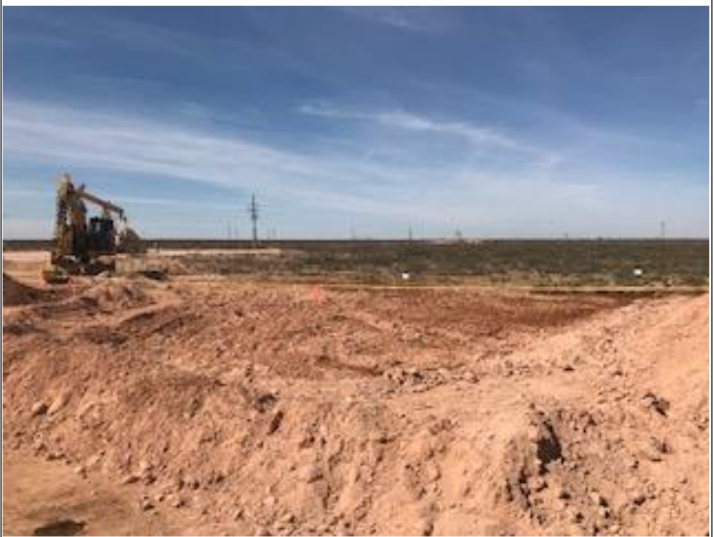
Southwestern view of the final excavation extent.
