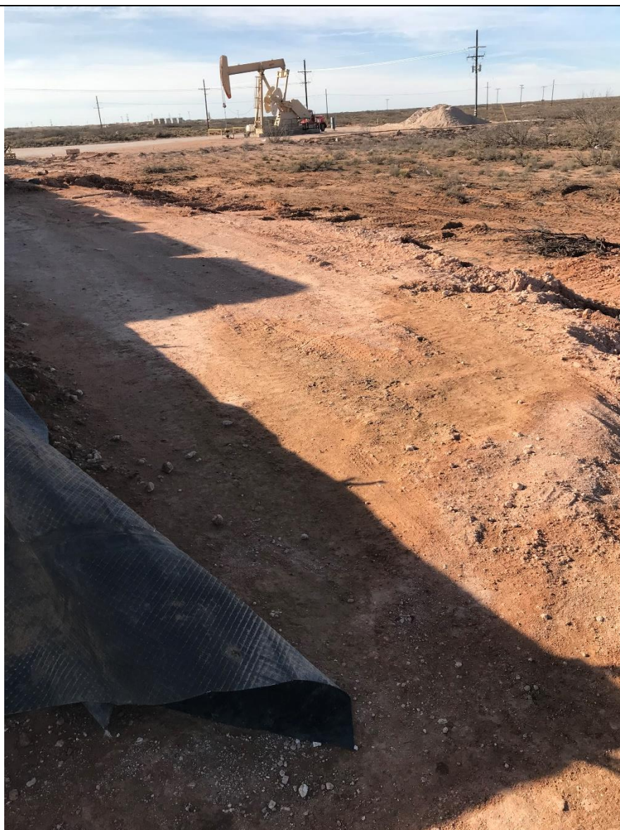
Southwestern view of the northern release area prior to excavation activities.
