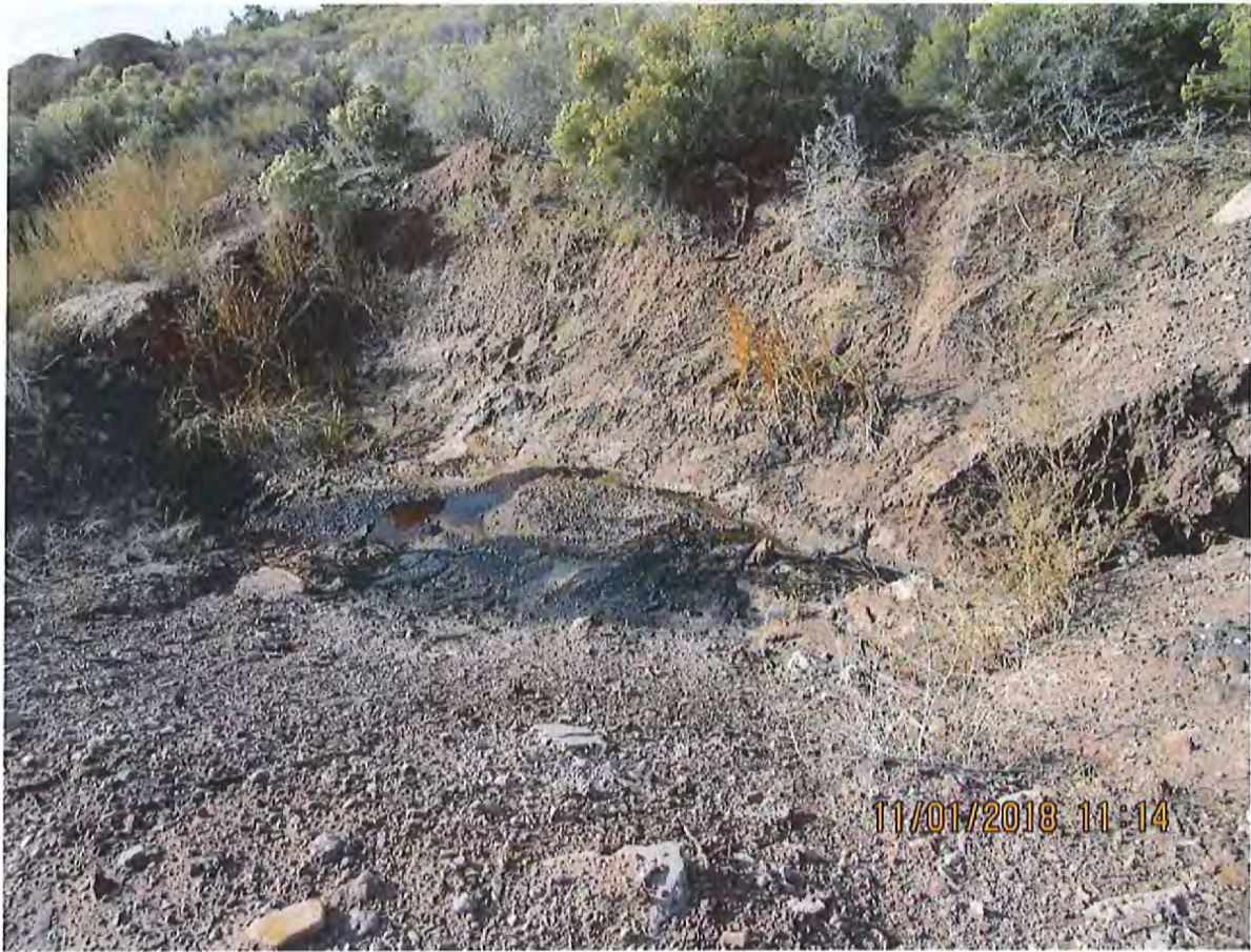
Photo No. 3 of location with concentrated discharge of hydrocarbons midway along retention ditch. Looking west, midway along retention ditch.
