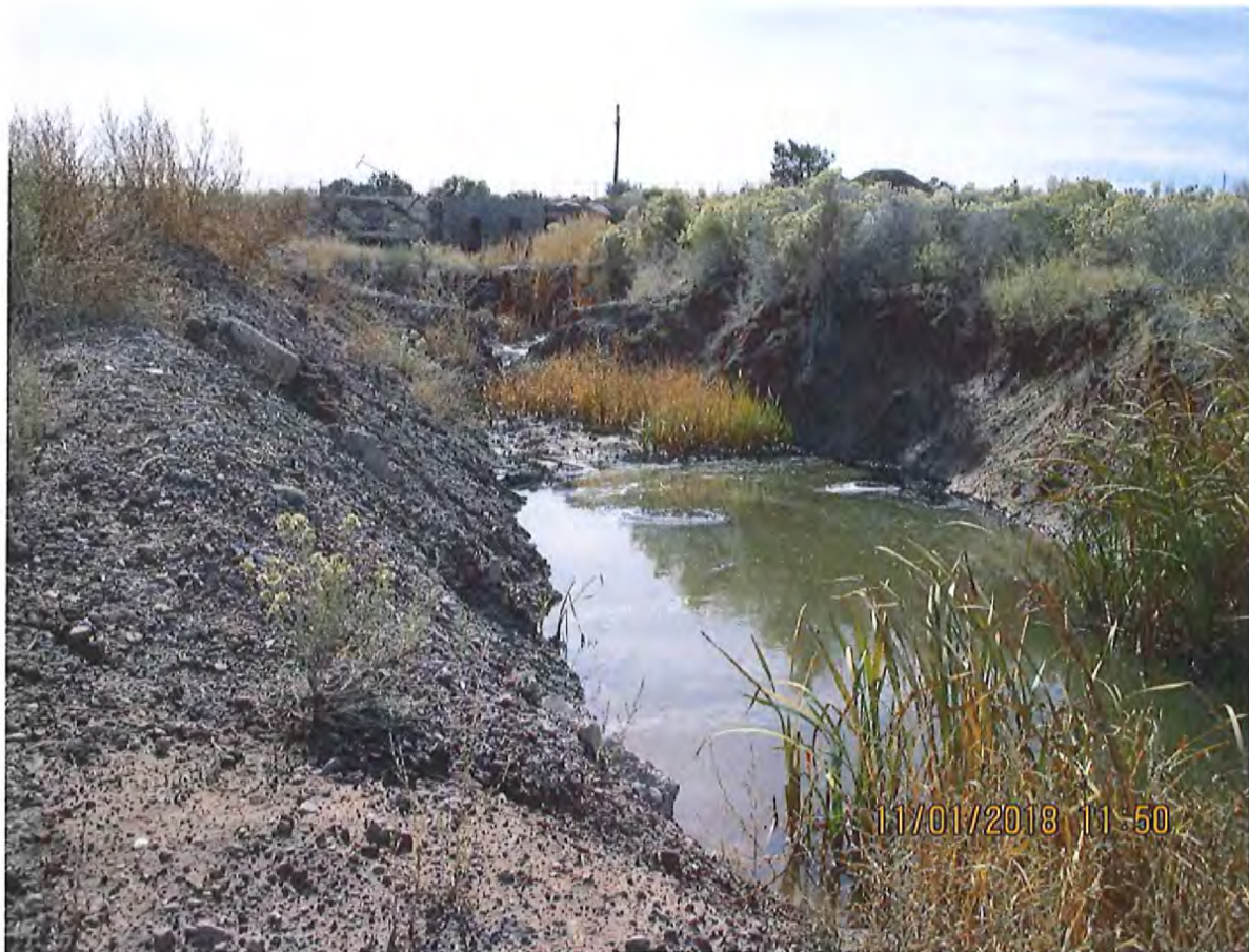
Photo No. 2: Looking south along retention ditch, midway between north and south ends. Some hydrocarbon staining along perimeter of ditch, but very little hydrocarbon present on water. Location of concentrated hydrocarbon discharge at upper (southern) end of this ponded area.
