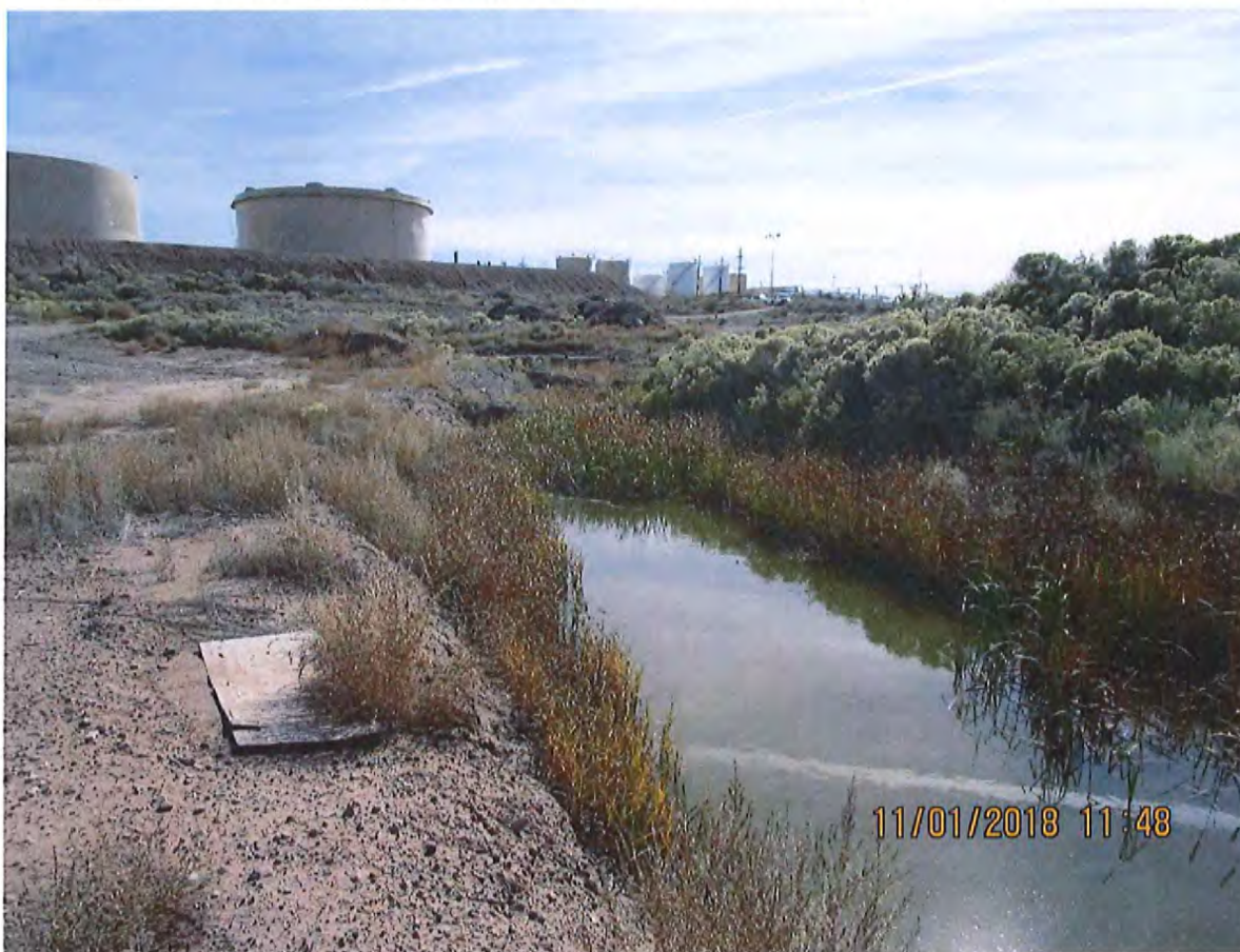
Photo No. 1 of lowermost (northern) end of retention ditch. Oil stained vegetation shown around edges of ditch but no recoverable product on water.
