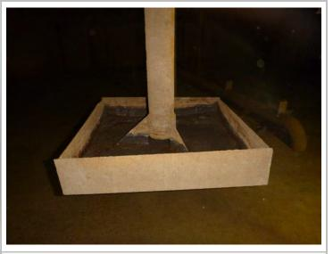
Old Style roof drains & catch pans (5) - no longer in use
