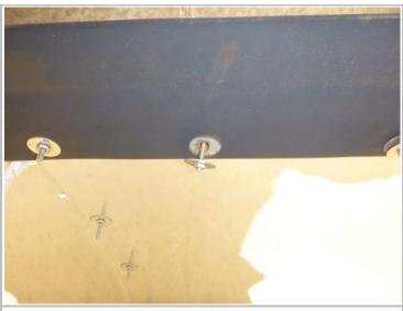
Roof Seal - loose and missing hardware.
