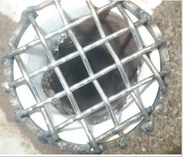
Roof vent/emergency drain - has screen but open to rain- see recommendations
