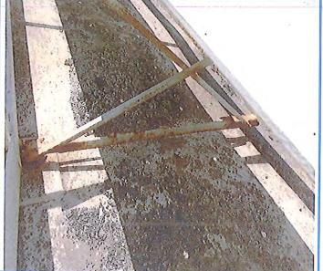
Corrosion and coating failure on roof platform support
