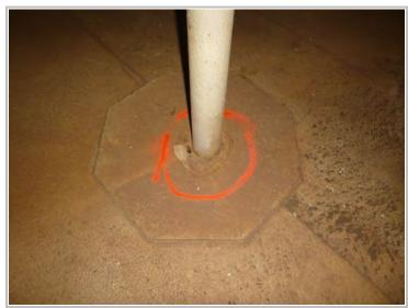
Striker Pates (3) – corrosion up to 0.140" in depth, install new pad over old
