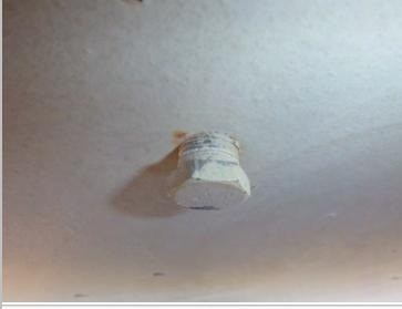
3/8" threaded plugs in shell – plugs not seal welded
