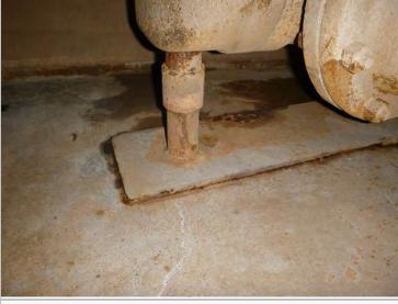
Swing Joint (Suction Line) - Support not seal welded
