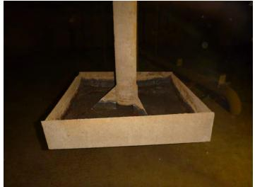
Old Style roof drains & catch pans (5) - no longer in use
