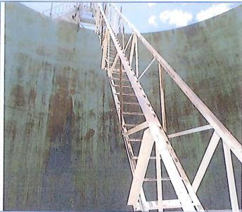
Coating failure on ladder and inside of shell
