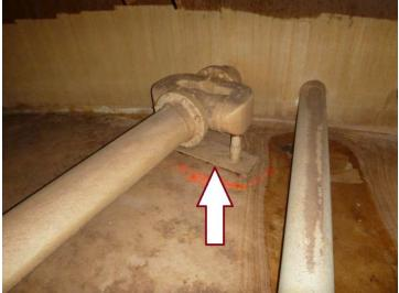
Piping Knuckle/Inlet "Y" - Pads under support are stitch welded.
