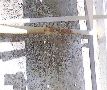
Corrosion and coating failure on roof platform support
