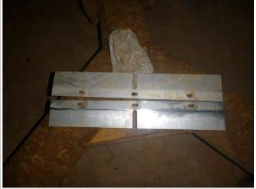
Roof Seal - loose and missing hardware.
