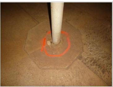
Striker Pates (3) – corrosion up to 0.140" in depth
