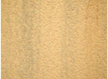
Shell  $2^{nd}$  course and above – complete coating failure; 0.20" to 0.040" general corrosion/pitting
