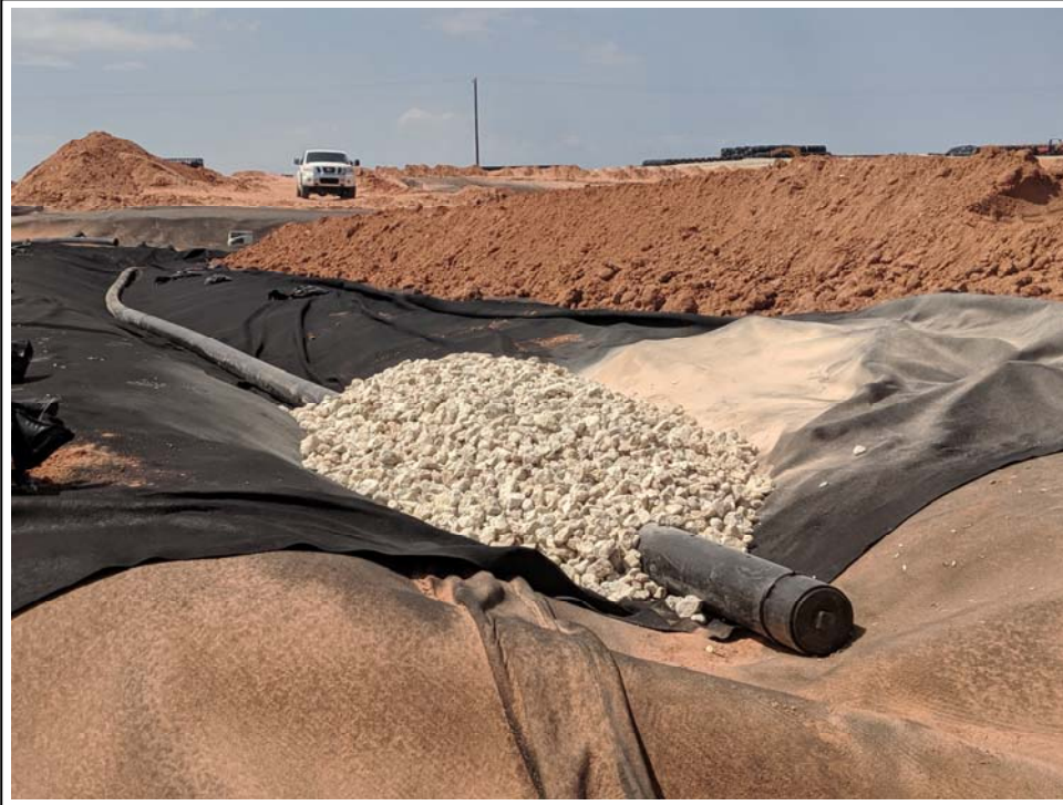
23. 5/29/2019: Select aggregate placement and leachate collection pipe end cap (view to south)
