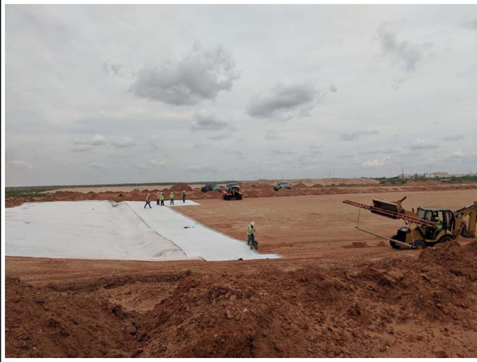
7. 5/7/2019: Deployment of GCL panels along west edge of Area B (view to north)
