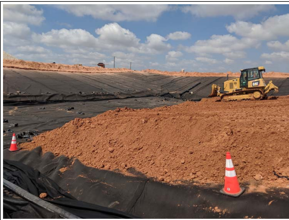
28. 5/29/2019: Operators use cones as guides to ensure 2-foot minimum thickness (view to west)
