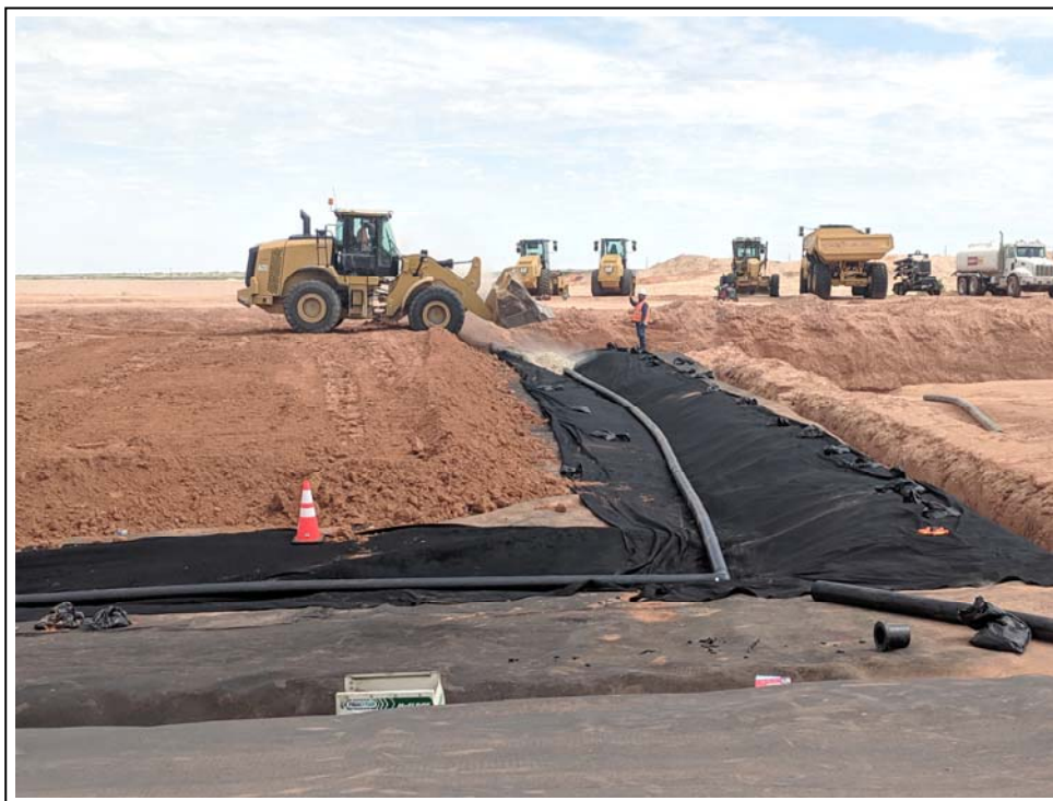
21. 5/29/2019: Placement of select aggregate on nonwoven geotextile fabric (view to north)
