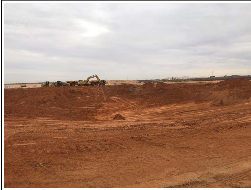
1. 3/7/2019: Initial excavation of subgrade from existing soil stockpiles (view to east)
