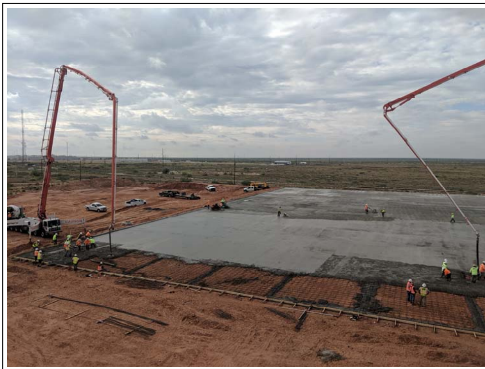
40. 9/10/2019: Operation of two pumps for placement of Area A pad (view to south)
