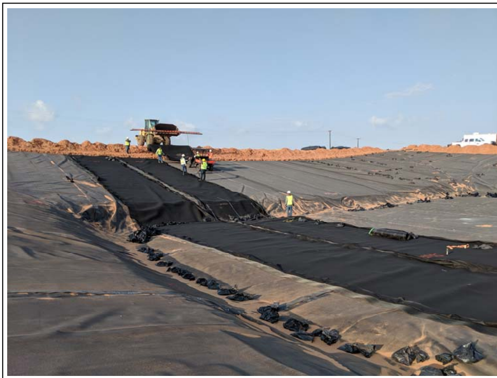
16. 5/11/2019: Deployment of 200-mil geonet panels along Area C slope (view to southwest)
