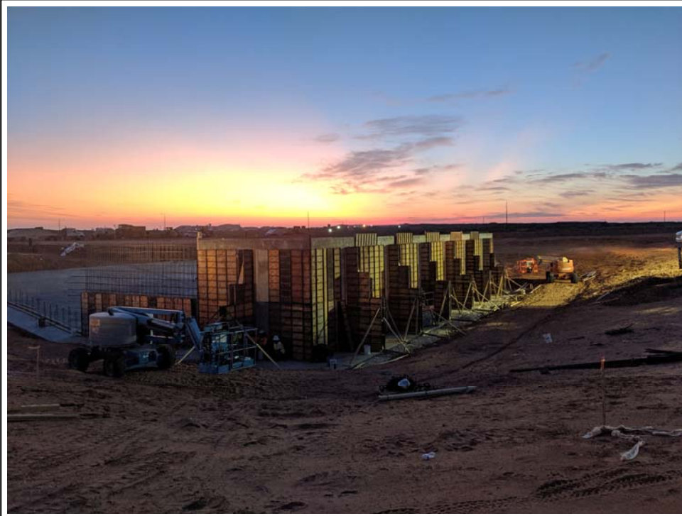
41. 8/29/2019: Wall forms and counterforks along south wall of Area C sump (view to southwest)
