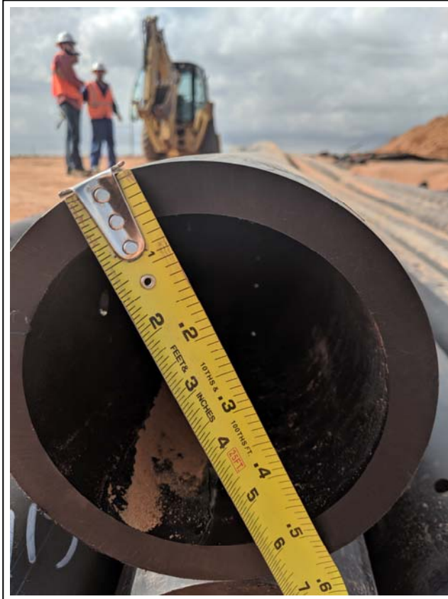
19. 5/29/2019: Diameter of 6-inch perforated SDR 11 HDPE pipe, 40 feet
