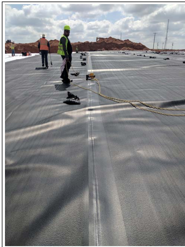
12. 6/1/2019: Fusion weld along 60-mil geomembrane, Area A (view to east)
