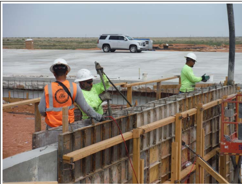
42. 8/24/2019: MHAT crews vibrating each lift of concrete during placement (view to northwest)
