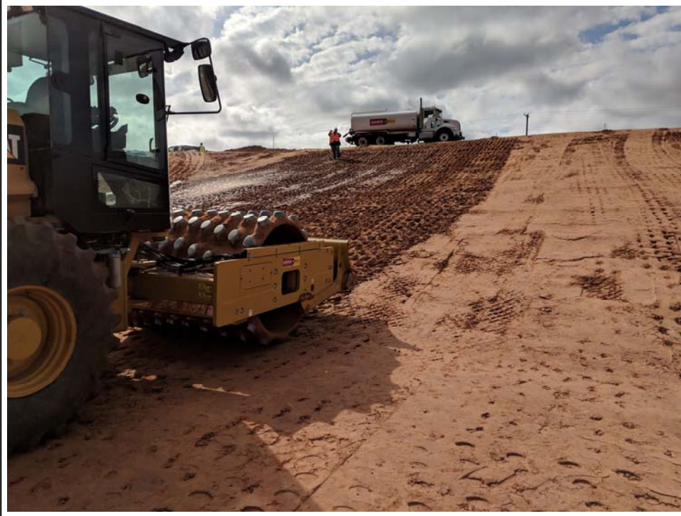
3. 3/22/2019: Sheepfoot and water on south slope of sump (view to southeast)
