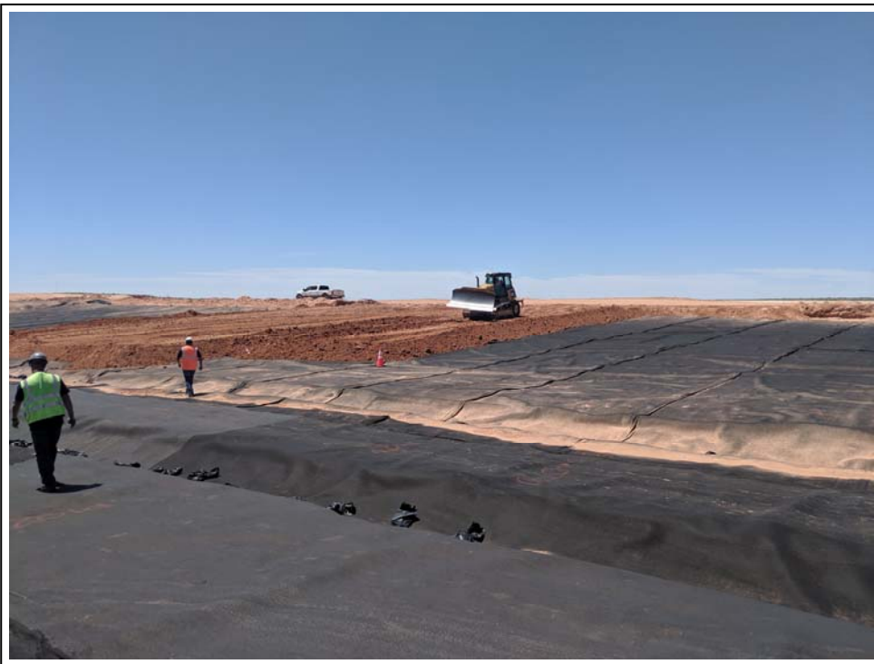
26. 5/28/2019: Pushing backfill to grade (view to northwest)
