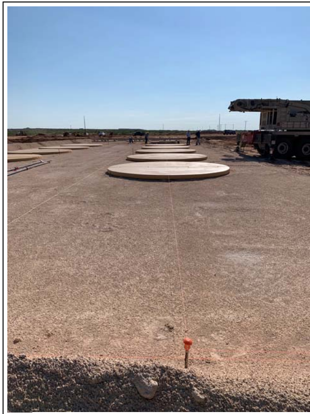
48. 9/4/2019: Placement of polyurethane tank pads (view to east)
