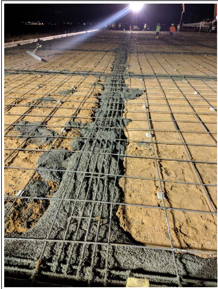
35. 9/9/2019: Pouring concrete footings on south end of pad (view to west)
