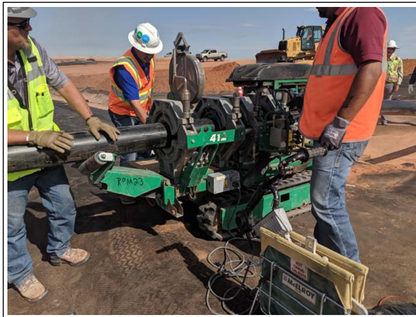
20. 5/29/2019: Fusion of HDPE leachate collection lines
