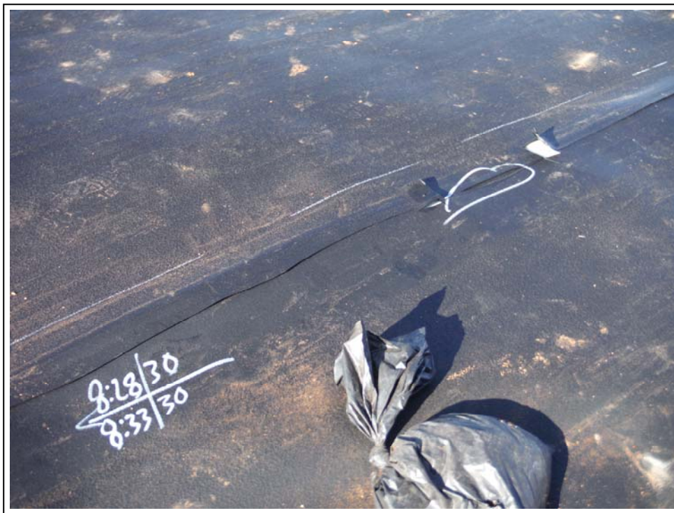
14. 6/11/2019: Location of seam pressure test and results
