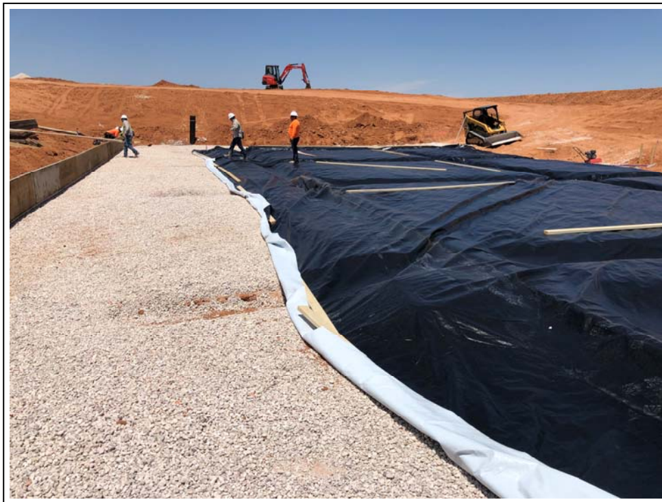
30. 6/26/2019: Placement of base aggregate and base liner in preparation of concrete, Area C (view to west)
