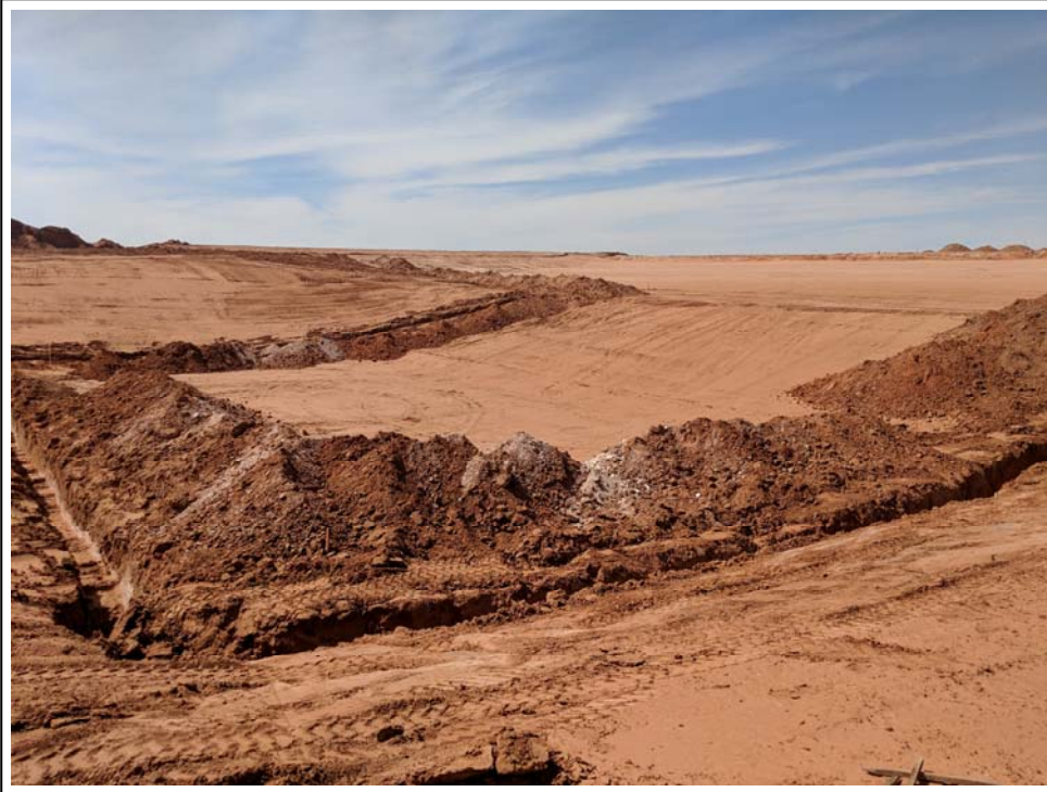
6. 4/4/2019: Mud jet out and sump (Areas B and C), leachate collection trenches (view to west)
