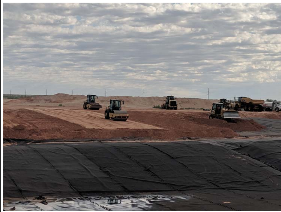
27. 5/29/2019: Compaction and placement of protective soil layer, Area B (view to north)
