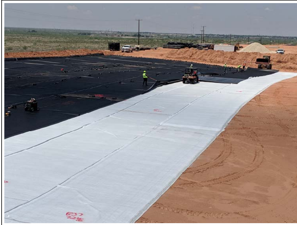
13. 6/1/2019: Deployment of 60-mil geomembrane, Area A (view to west)
