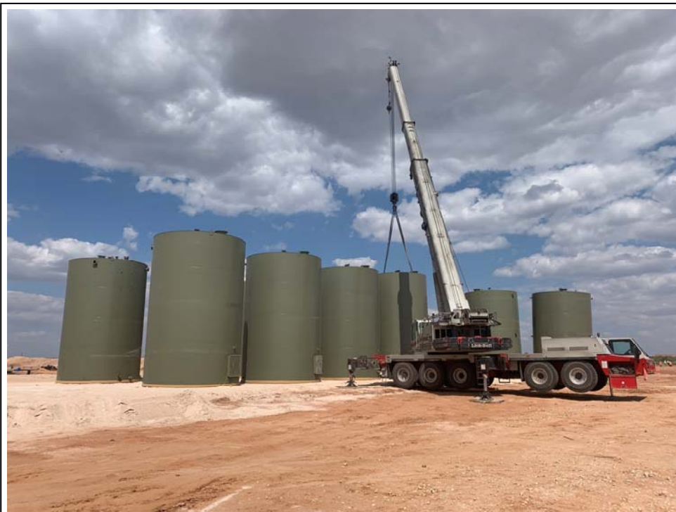
50. 9/4/2019: Crane lifting tanks onto pads in Area D (view to southwest)
