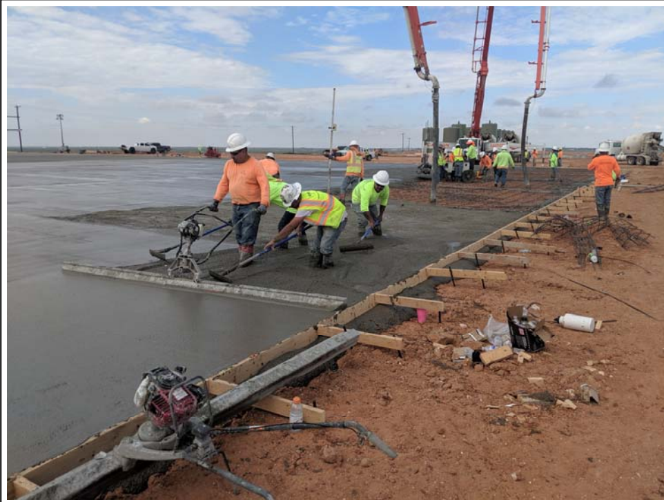
37. 9/10/2019: Vibrating screed operation along north end of Area A pad (view to west)
