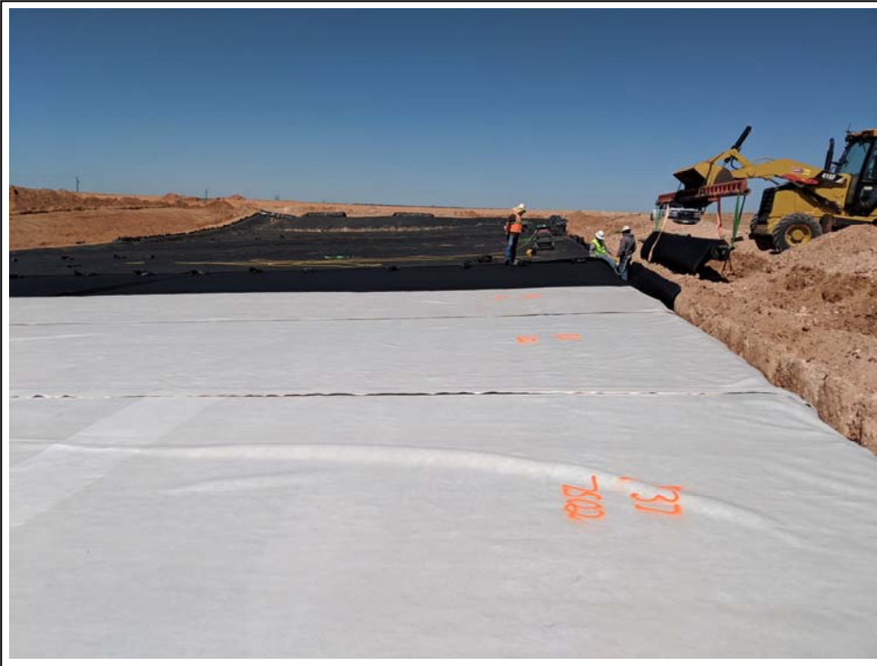
8. 5/8/2019: Mud jet out (Area B), deployment of GCL panels ahead of geomembrane liner (view to west)
