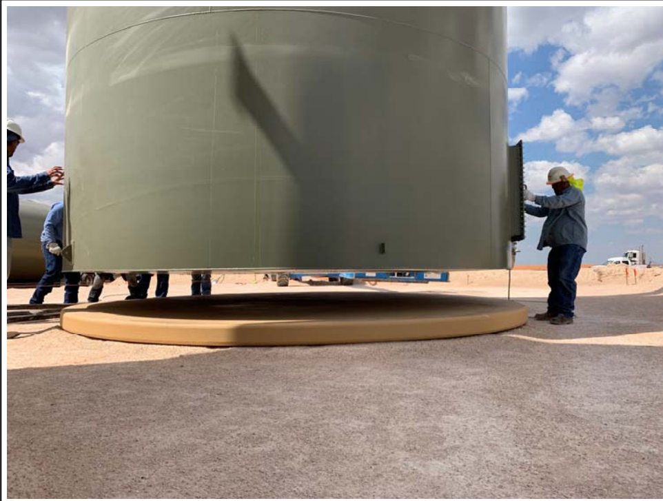
49. 9/4/2019: Lining up tank onto tank base
