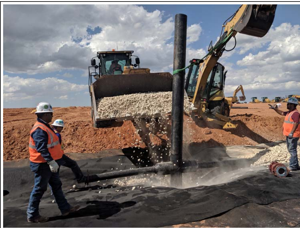
24. 5/29/2019: Installation of leachate collection standpipe for mud jet out (Area B) (view to north)
