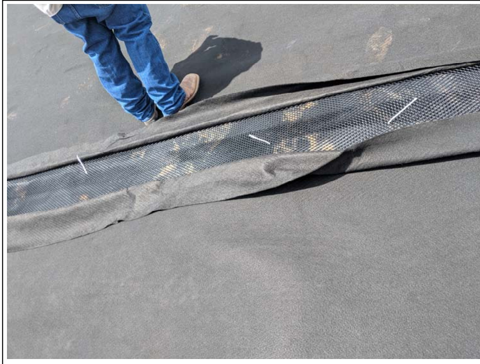
17. 5/11/2019: Zip ties used to tie panels together before fabric is seamed with welder and heat guns
