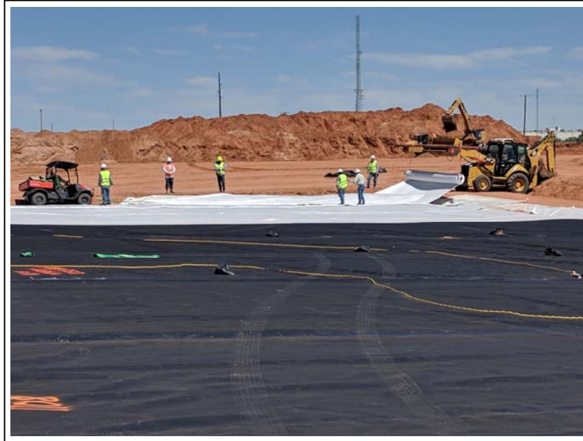
9. 5/8/2019: Mud jet out (Area B), deployment of GCL panels along east anchor trench (view to east)
