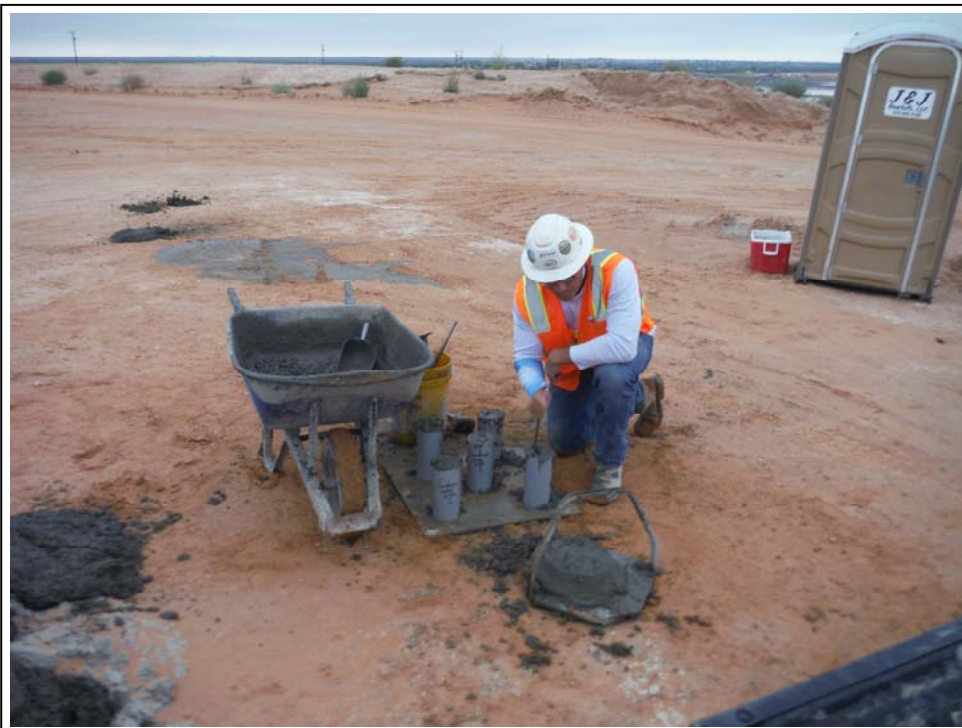
44. 8/28/2019: Beyond Engineering filling cylinders with concrete for geotechnical testing (view to southwest)
