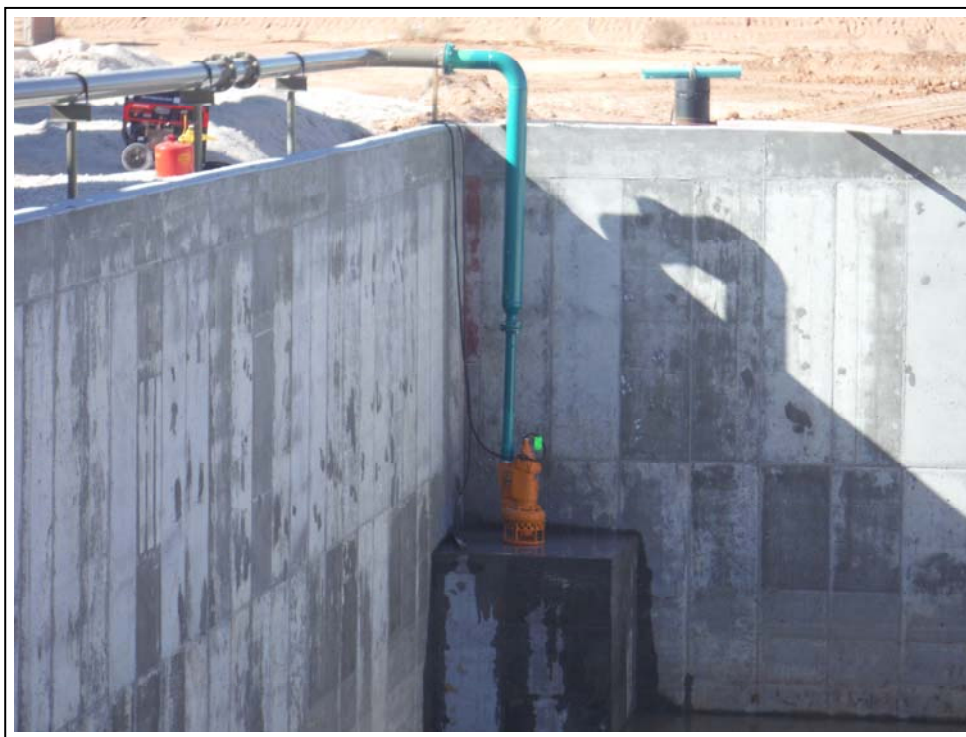
53. Pump installed on concrete stand in Area C sump that supplies water to processing tanks (view to west)
