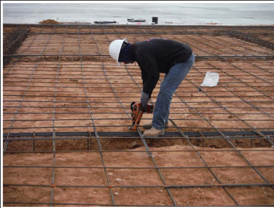
33. 11/12/2019: Using cordless rebar tying tool, Area A
