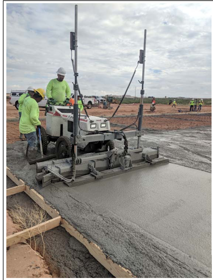
36. 9/10/2019: Operating the vibrating auto-screed to establish concrete grading (view to east)
