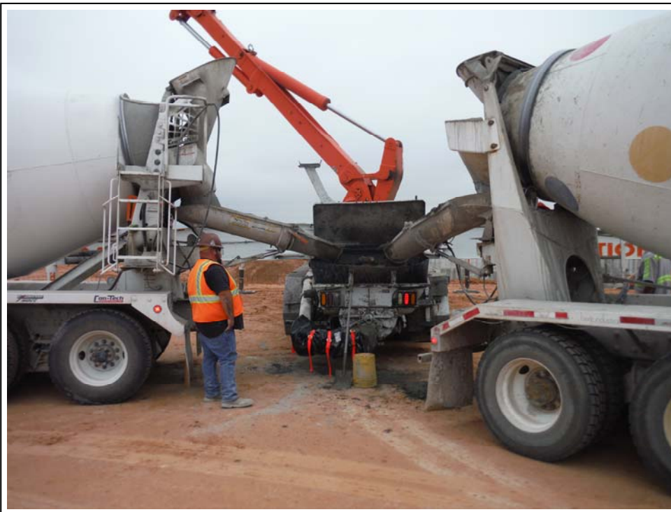
34. 8/28/2019: Discharging concrete into pump truck hopper (view to south)
