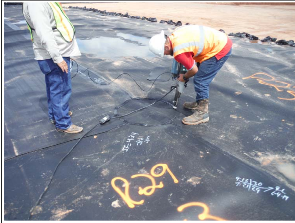
15. 6/11/2019: Extrusion welding patch over line, Area A
