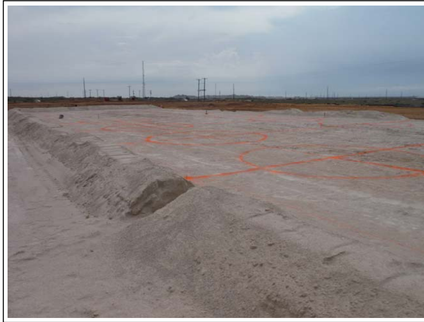
47. 8/28/2019: Area D markings for aboveground tank placement on crushed caliche pad (view to southeast)
