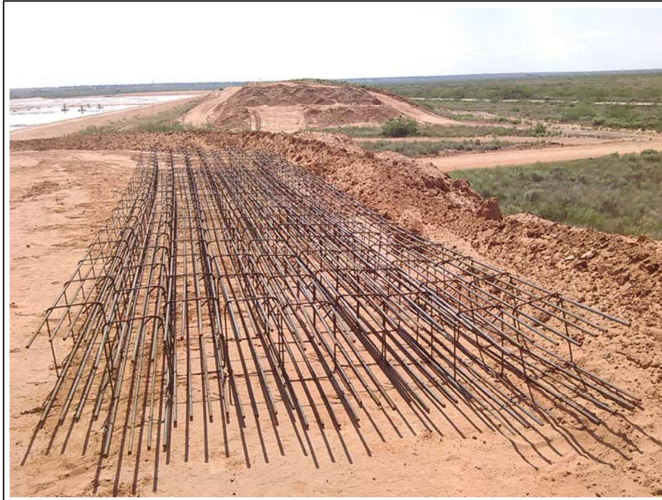
29. 6/18/2019: 40-foot tied rebar cages for footings
