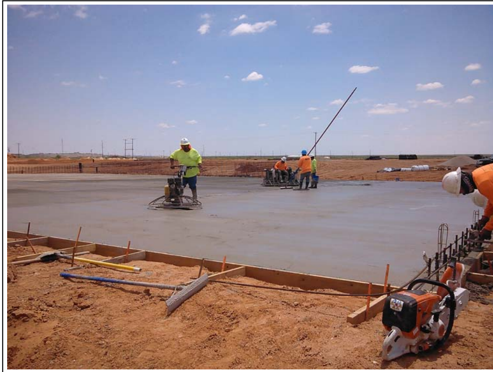
39. 7/24/2019: Power trowel finishing on west Area B pad (view to south)
