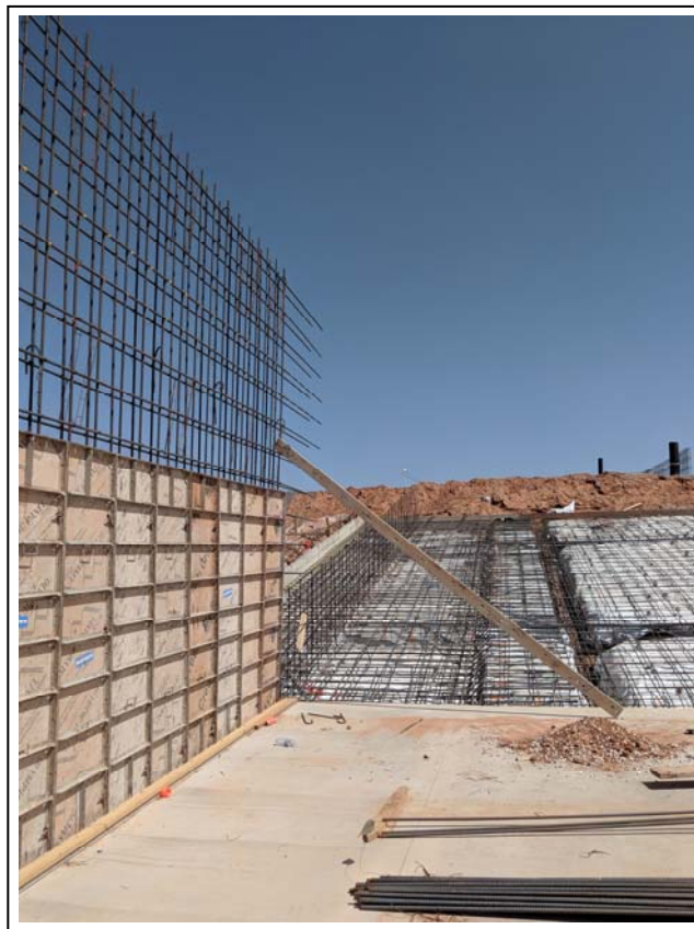
32. 8/1/2019: Rebar and lining placed on 19% grade to sump, construction of sump walls (view to north)
