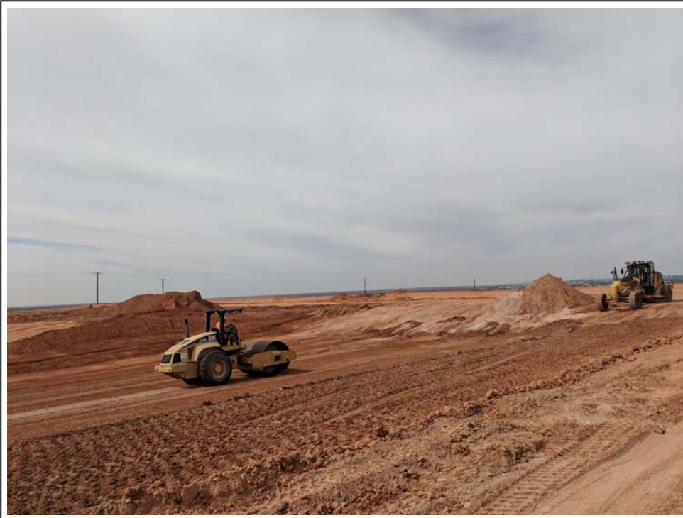
4. 3/28/2019: Mud jet out (Area B), grader and roller compaction (view to southwest)
