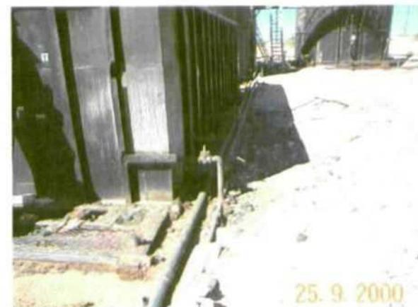
Photo 6 Stained soil from leaks or overflow. Some clean caliche fill brought in.
