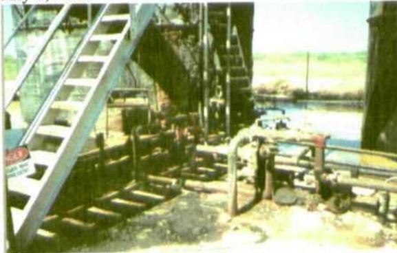
Photo 19 Standing fluid between tanks
