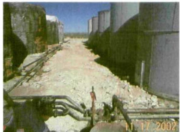
Photo 6. Area between tanks backfilled with clean soil.
