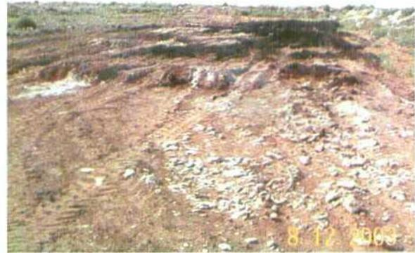
Photo 4: Cell 1 is full. Soil has been spread to approximately 8-inch thickness. Cell contains soils removed from excavations around tanks.
