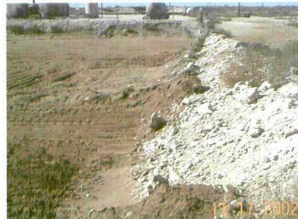
Photo 23. Contaminated soils in the landfarm are pushed up on the side of the berm.
