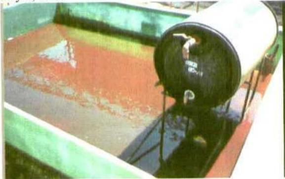
Photo 25 Drum secondary containment contains several inches of fluid.
