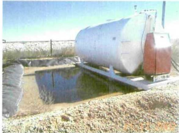
Photo 16. Fuel tank labeled and contained within a lined berm. Rainwater from recent rain event.
