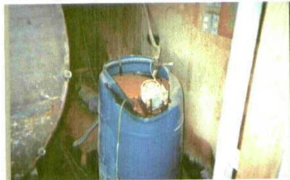
Photo 24 Barrel in boiler room is very full and does not have secondary containment.
