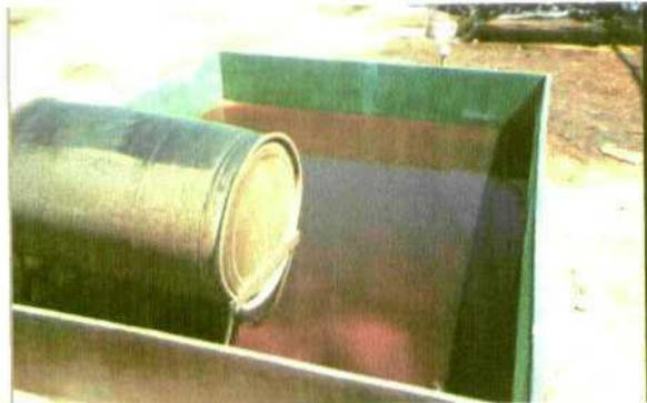
Photo 26 Drum secondary containment contains several inches of fluid.
