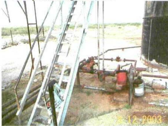
Photo 1: Insulated tank removed from SE corner of facility. Contaminated soils excavated and removed to landfarm.
