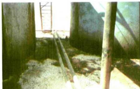
Photo 8      Leaks and spills between tanks
