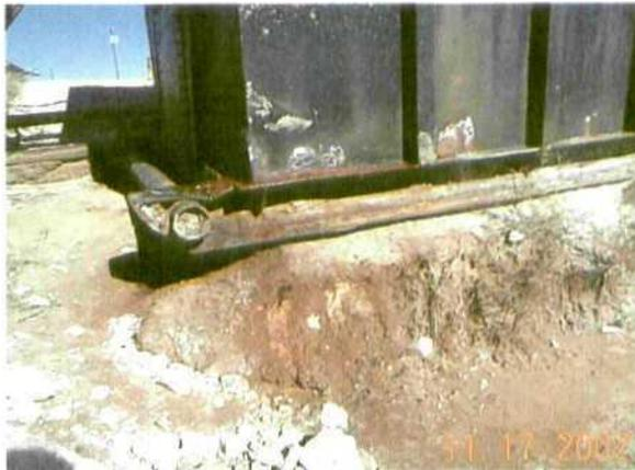
Photo 8. Parifin Tank is leaking a steady drip. The ground is very saturated with produced water.
