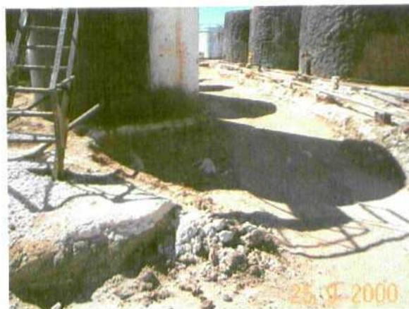
Photo 17 Area between tanks excavated and filled with clean fill.
