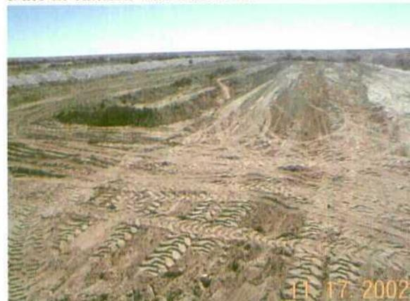
Photo 22. Contaminated soil piles within the landfarm have not been spread. Soil appear to be compacted and not turned.
