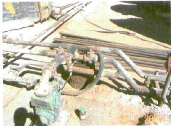
Photo 11 Valve catchment shows numerous overflows.
