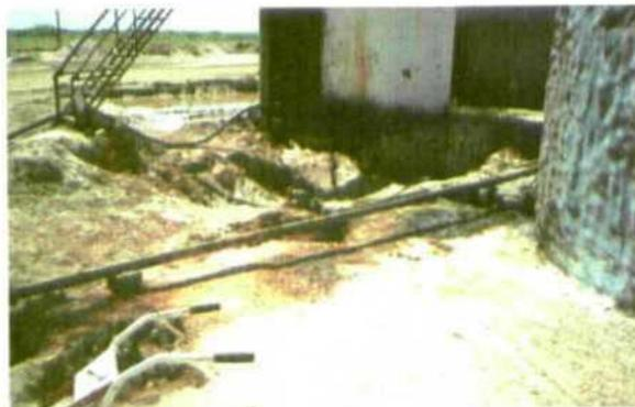
Photo 10      Liquid ponded around tanks
