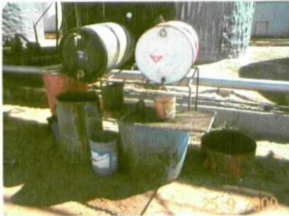
Photo 1 Chemical containers with valve catchments.
