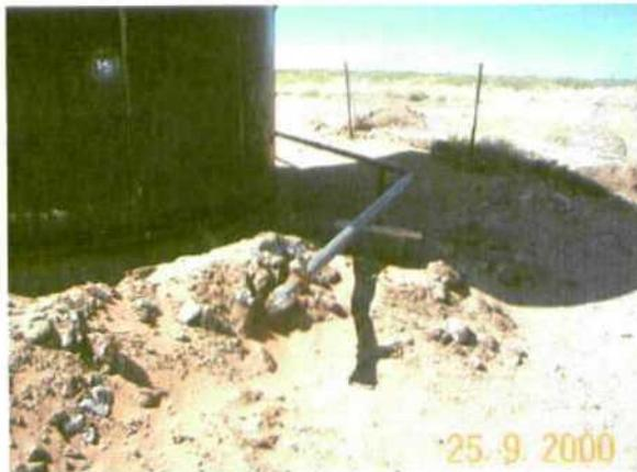
Photo 9 Valve with out catchment. Berm is low.
