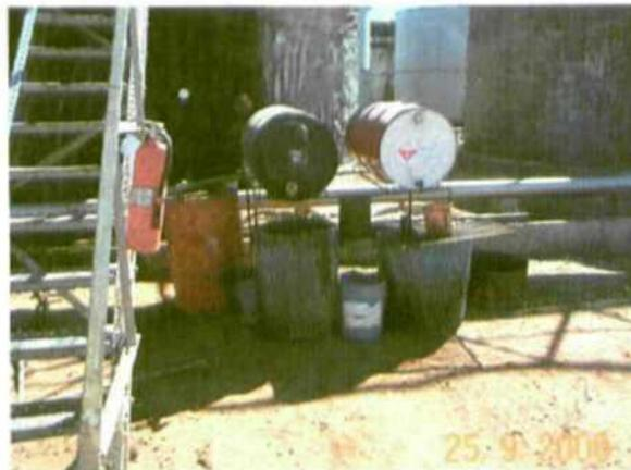
Photo 2 Chemical containers with valve catchments.
