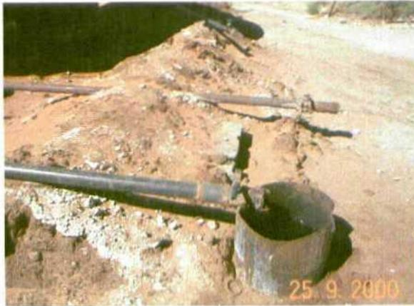
Photo 8 Valve catchment 1/2 full. Stained soil from spills and overflows
