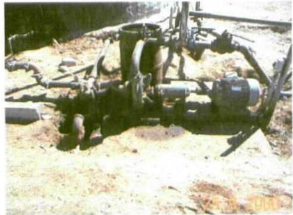
Photo 4 Stained soil from leaks or overflow of full drum.
