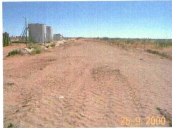
Photo 21 Contaminated soil spread south of fence line. Landfarm area not bermed or secured within fence.
