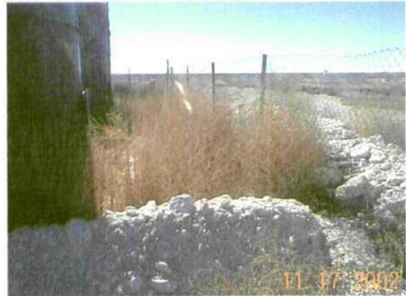
Photo 10. Berm around the outside of the facility fence and around the tanks in the southwest corner.
