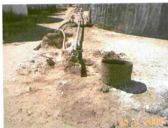
Photo 18 Stained soil from spills and leaks. Catchment not under the valve.
