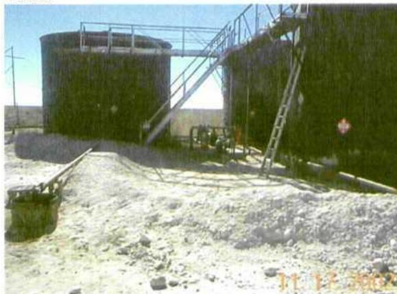
Photo 9. Tanks in the southwest corner are bermed and labeled.
