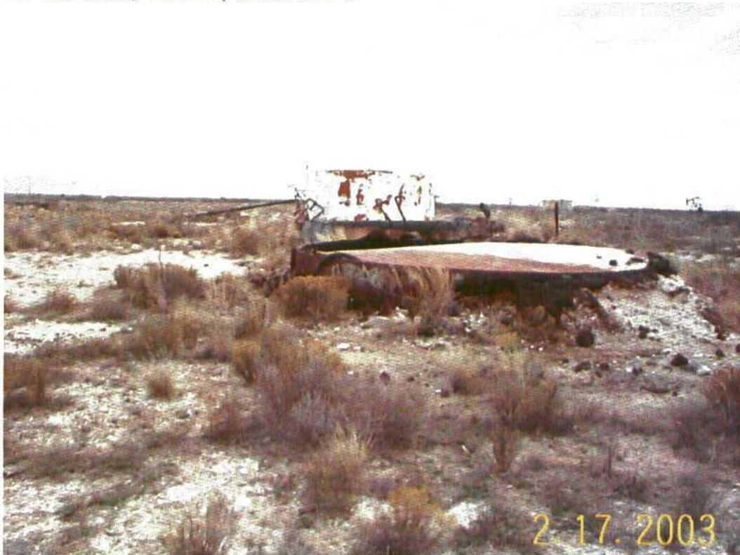
Photo 1. 2-250 bbl Buried slop tanks containing paraffin and some water and 1-250 bbl orange foam insulated tank contents unknown. Looking East
