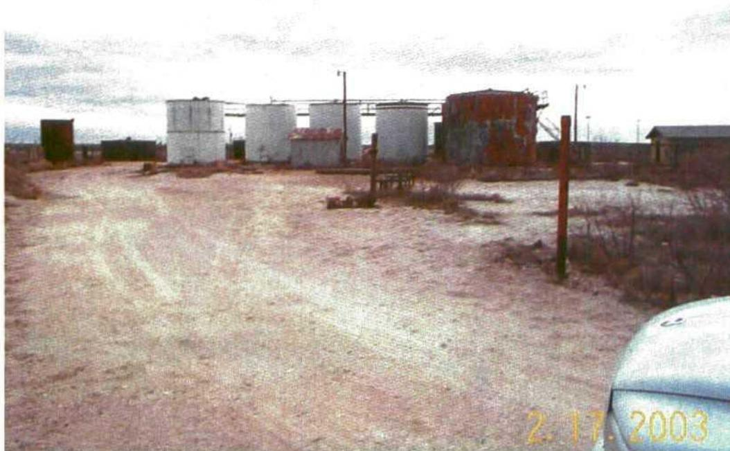
Photo 12. From left to right, 1-210 bbl welded tank, 1-250 bbl bolted tank, 1-500 bbl bolted tank, 3-500 bbl welded tanks, 10'x10' shed, 2-750 foam insulated tanks, enclosed LACT unit and 2'x30' shed. Looking east.
