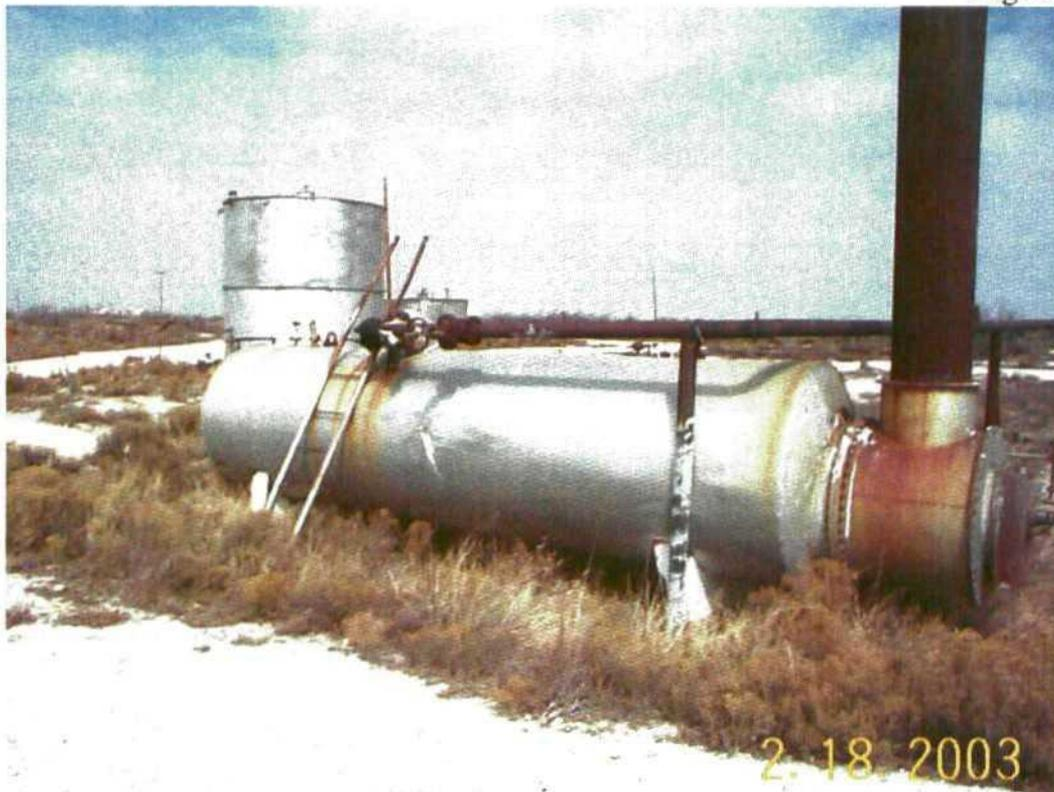
Photo 11. From the foreground to the background. One 6'x20' horizontal heater, 1-500 bbl bolted tank with 5' of material and 1-250 bbl bolted tank with 4' of material. Looking northeast.
