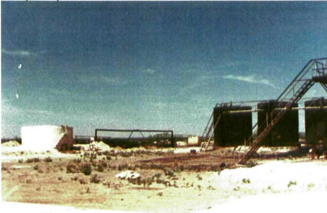
Photo 1. Operations on the south side of the road. 1-250 bbl insulated tank, 2-250 bbl buried tanks, 3-500 bbl foam insulated tanks Looking southwest. (This photo was taken before the cat walks were removed.)
