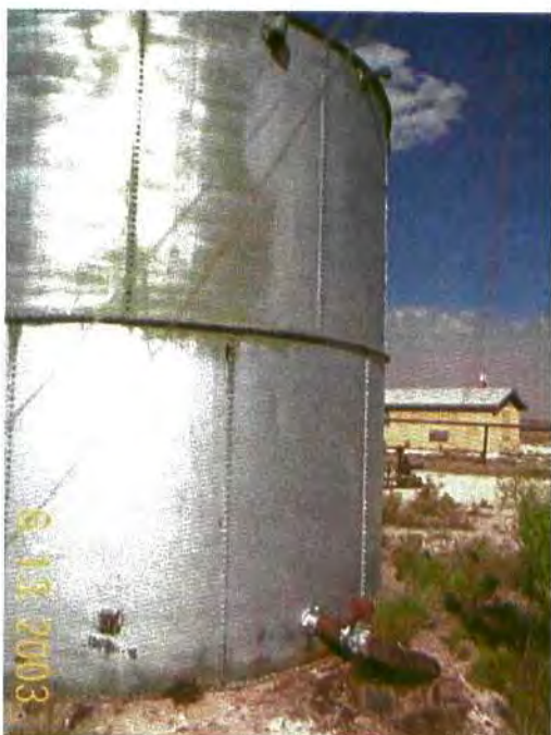
Photo 15. High 500 bbl tank with 5 feet of material. Looking east.
