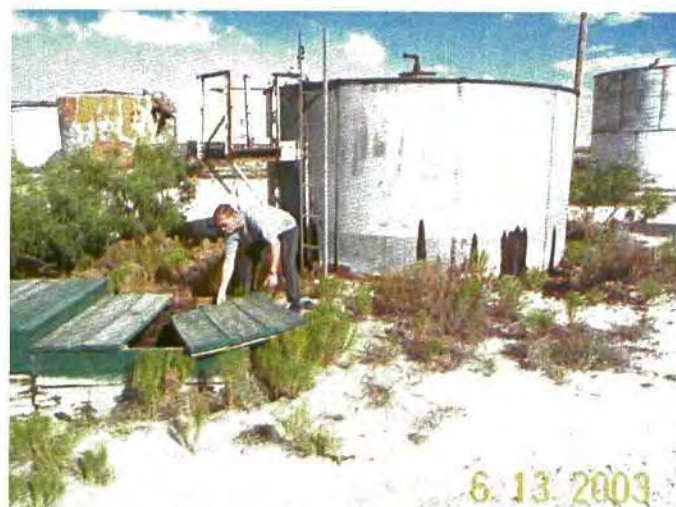
Photo 17. Leaking low 250 bbl tank and cellar. Looking east.
