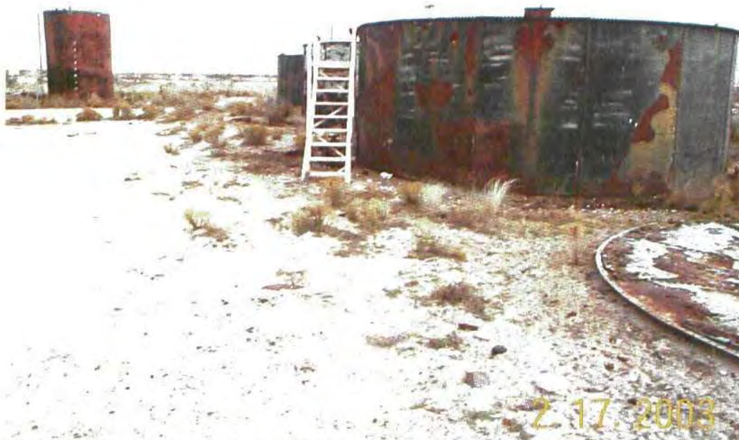
Photo 9. From left to right, 1-210 bbl welded tank and 3-250 bbl bolted tanks. Looking north.
