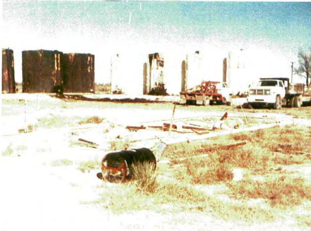
Photo 2. South side 7-500 bbl tanks insulated. Concrete footing frame. Looking northwest. (This photo was taken after the catwalks were removed.)
