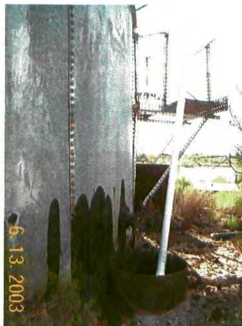
Photo 16. Leaking low 250 bbl tank with 4 feet of material. Looking west.
