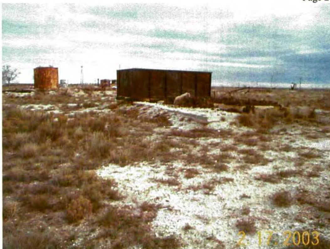
Photo 3. 36x20 concrete pad with dried parifin piles on pad. Steele plate box 8'h x 20'w x 10'l set on north end of concrete. Looking north-northeast
