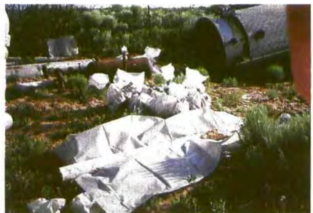
Pipe laid on polyethylene to be wrapped and sealed.
