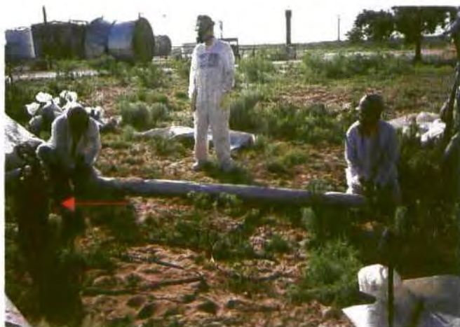
Pipe wrapped and being sealed. The sprayer (arrow) contains water to wet the asbestos when it is being removed.
