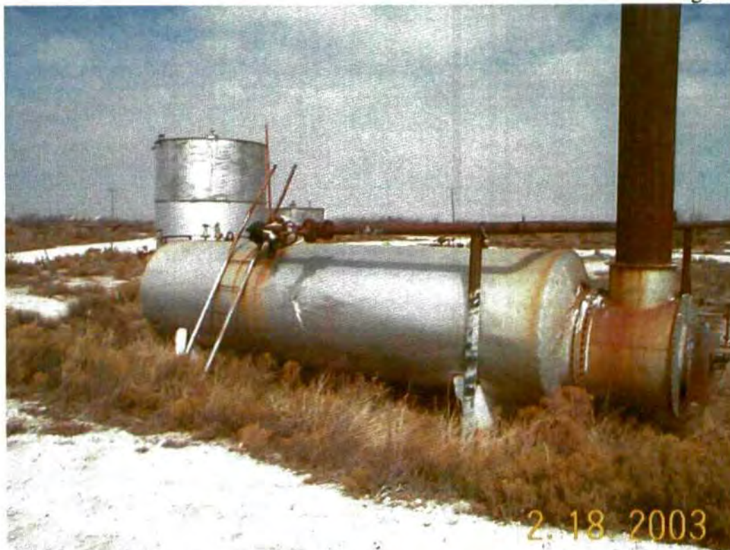
Photo 11. From the foreground to the background. One 6'x20' horizontal heater, 1x 500 bbl bolted tank with 5' of material and 1-250 bbl bolted tank with 4' of material. Looking northeast.
