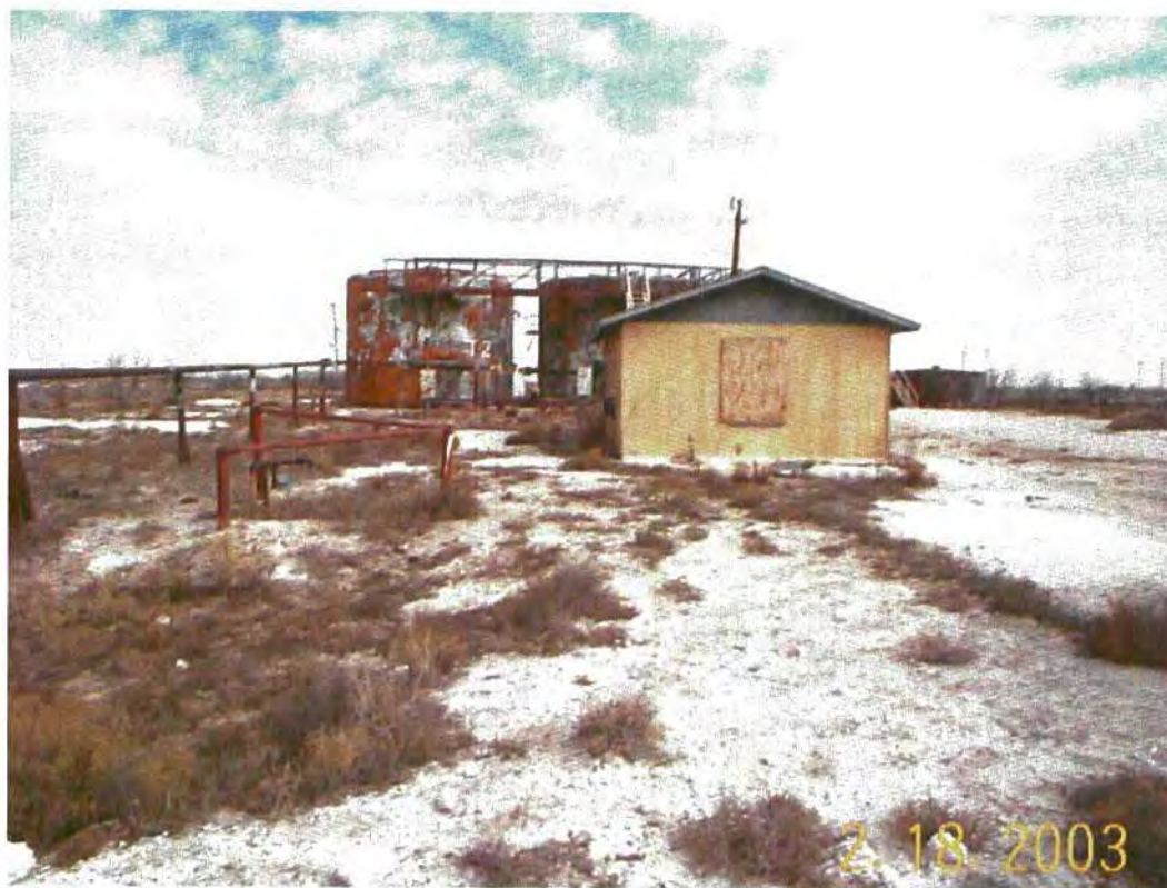
Photo 10. From left to right, 2-750 bbl foam coated tanks, 20'x 30' office building and 1-250 bolted tank. Looking North.
