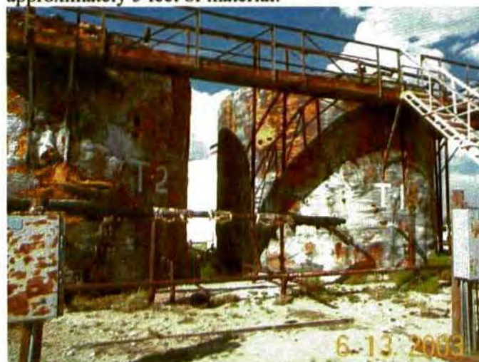
Photo 11. Two foam coated 750 or 1000 bbl tanks that are to be left.
