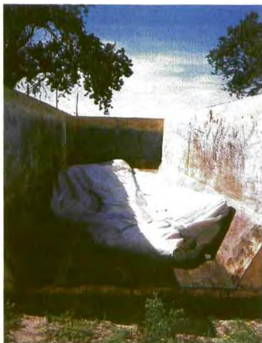
View of waste sealed in the polyethylene liner of the dumpster.
