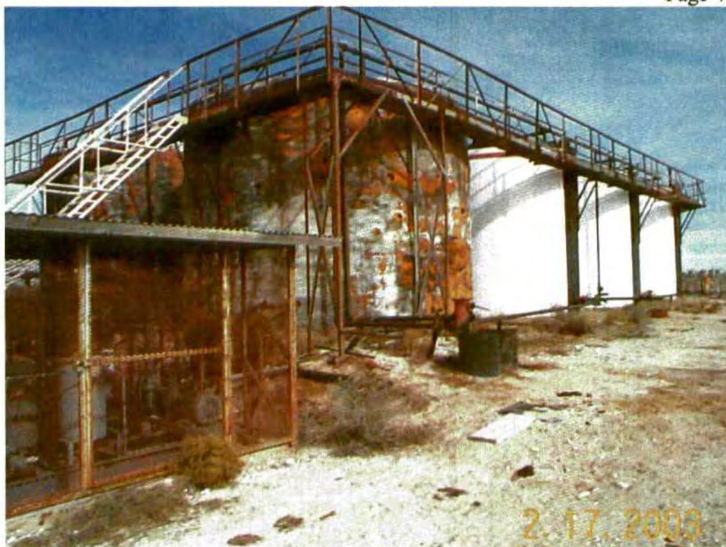
Photo 7. Enclosed lact unit, 2-750 bbl foam insulated tanks, 3-500 bbl welded tanks one additional 500 bbl bolted tank sits behind these and is accessible from the catwalk. Looking northwest
