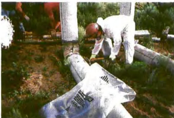
Preparing the area to remove insulation from an elbow that will be cut.
