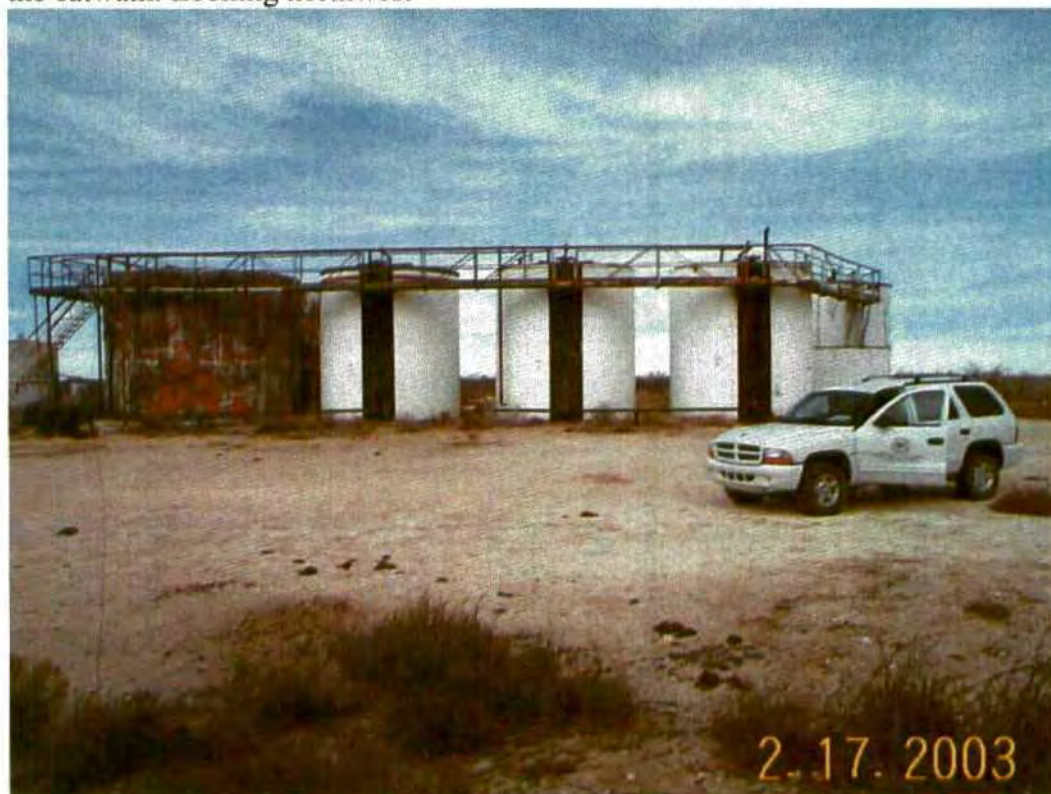
Photo 8. 2-750 bbl foam insulated tanks, 3-500 bbl welded tanks and 1-500 bbl bolted tank. Looking west.
