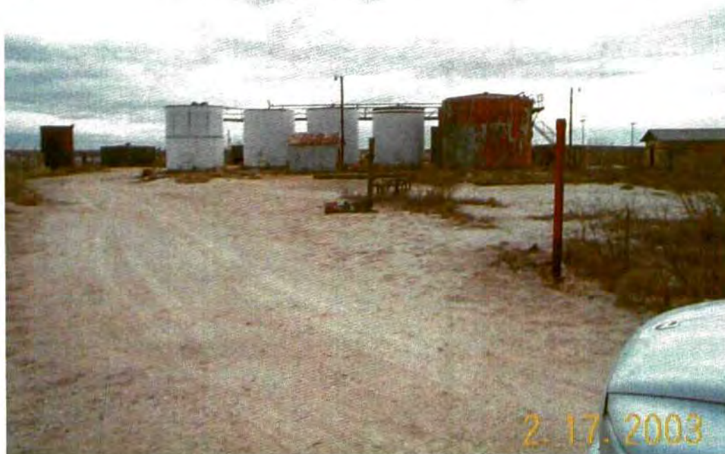
Photo 12. From left to right, 1x210 bbl welded tank, 1x250 bbl bolted tank, 1x500 bbl bolted tank, 3x500 bbl welded tanks, small shed, 2x750 foam insulated tanks, enclosed lact unit and 2'x30' shed. Looking east.
