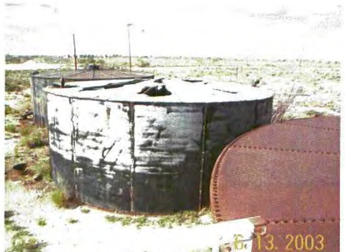
Photo 5. Three bolted 250 bbl tanks in the northeast corner of facility. Looking north-northeast.
