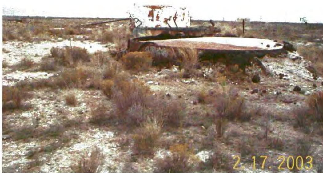
Photo 1. 2- Buried 250 bbl slop tanks containing Parifin and some water and one orange foam coated 250 bbl tank contents unknown. Looking East
