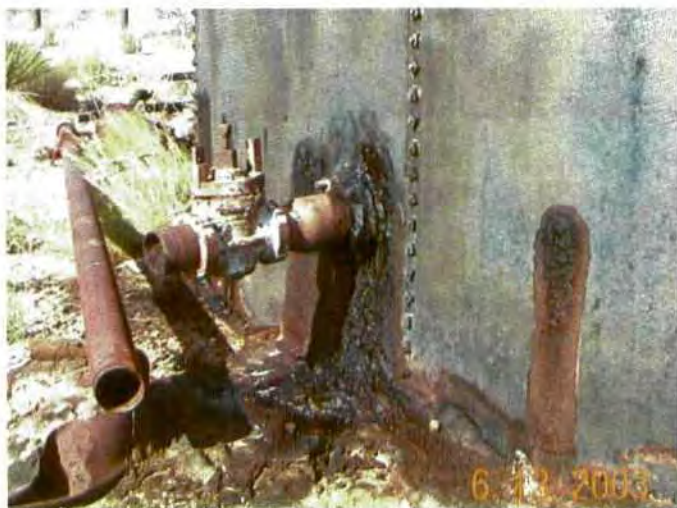
Photo 7. Leaking bolted tank.
