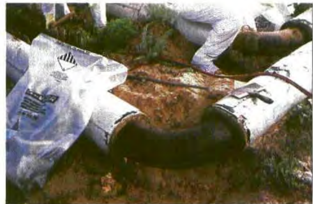
Cleaned elbow ready for cutting.
