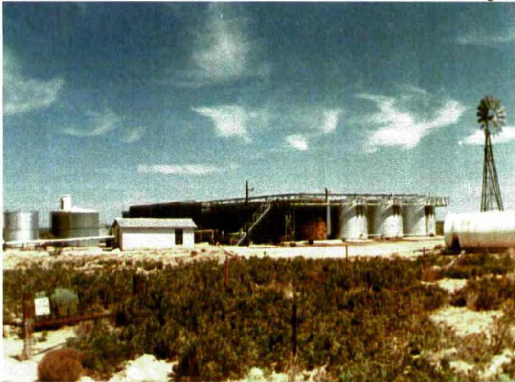
Photo 7. North side from left to right two tanks and vertical treater, office building, enclosed lact unit, 14-250 to 750 bbl bolted and welded tanks and foam insulated tanks, 1- fractank, windmill tower, Looking northwest.
