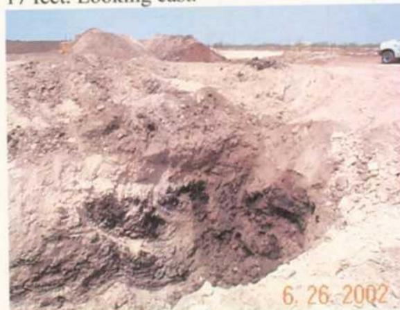
Photo 11. Pit 3 along south fence. Material was saturated with hydrocarbons. Looking northeast.
