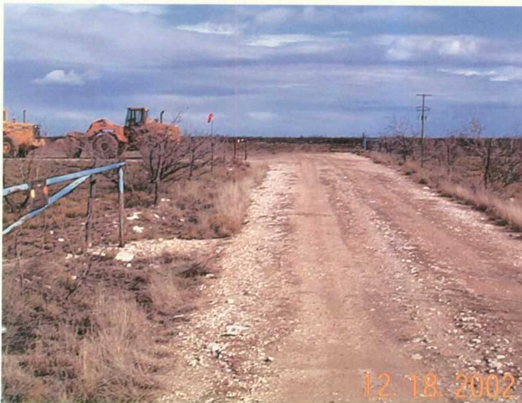
Photo 1: Goodwin Treating Plant entrance. Looking east. Remediation complete, excavations filled, and site compacted and mounded.
