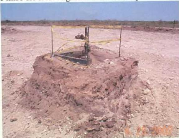
Photo 1. Wellhead left in place. Scheduled to be plugged in 2002. Looking northeast
