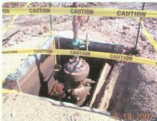
Photo 4. Wellhead. Pressure unknown. Advised contractor to excavate only around the outside of the wellhead.
