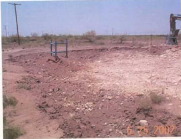
Photo 7. Excavation of the southwest corner of the facility. Overflows from south treater have been excavated beyond the fence line to the south and west.
