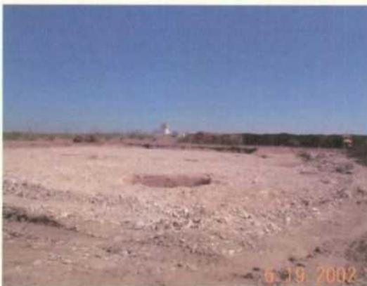
Photo 6. One of several holes dug for samples to be taken. GRO and DRO run on these holes and highest TPH was 183.7. Told contractor to backfill, as he was concerned that cattle may be lost in holes.
