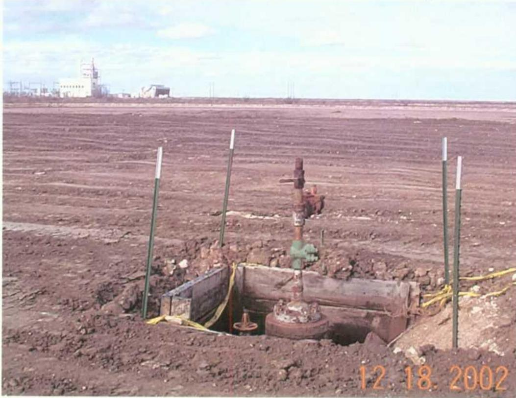
Photo 1: Agua Well at the Goodwin Treating Plant. Looking north-northwest. Remediation complete, excavations filled, and site compacted and mounded.
