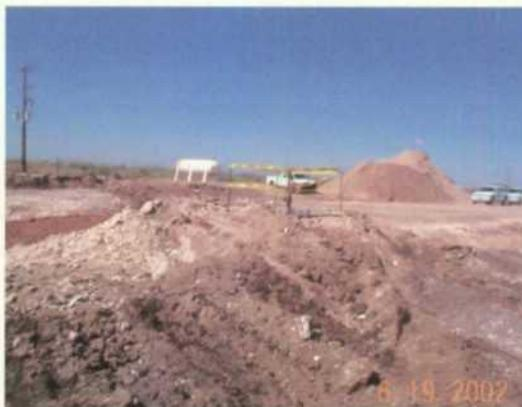
Photo 5. View #2 of wellhead. Contractor will only excavate this close to wellhead on all sides. Looking Southwest
