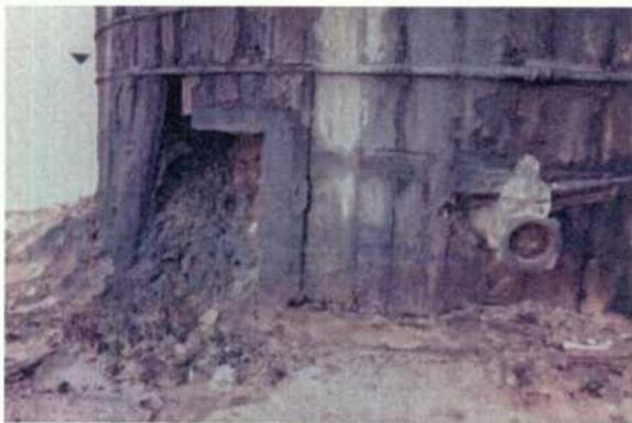
Entry for the north and south treaters was not possible during the initial investigation to determine the contents. The volume of hydrocarbon contaminated soils in the on site soil pile and around the tanks is estimated to be 1450 cubic yards.
