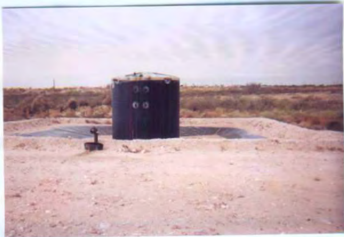
CATCH TANK for Loading Ramps & Wash Out pit.
