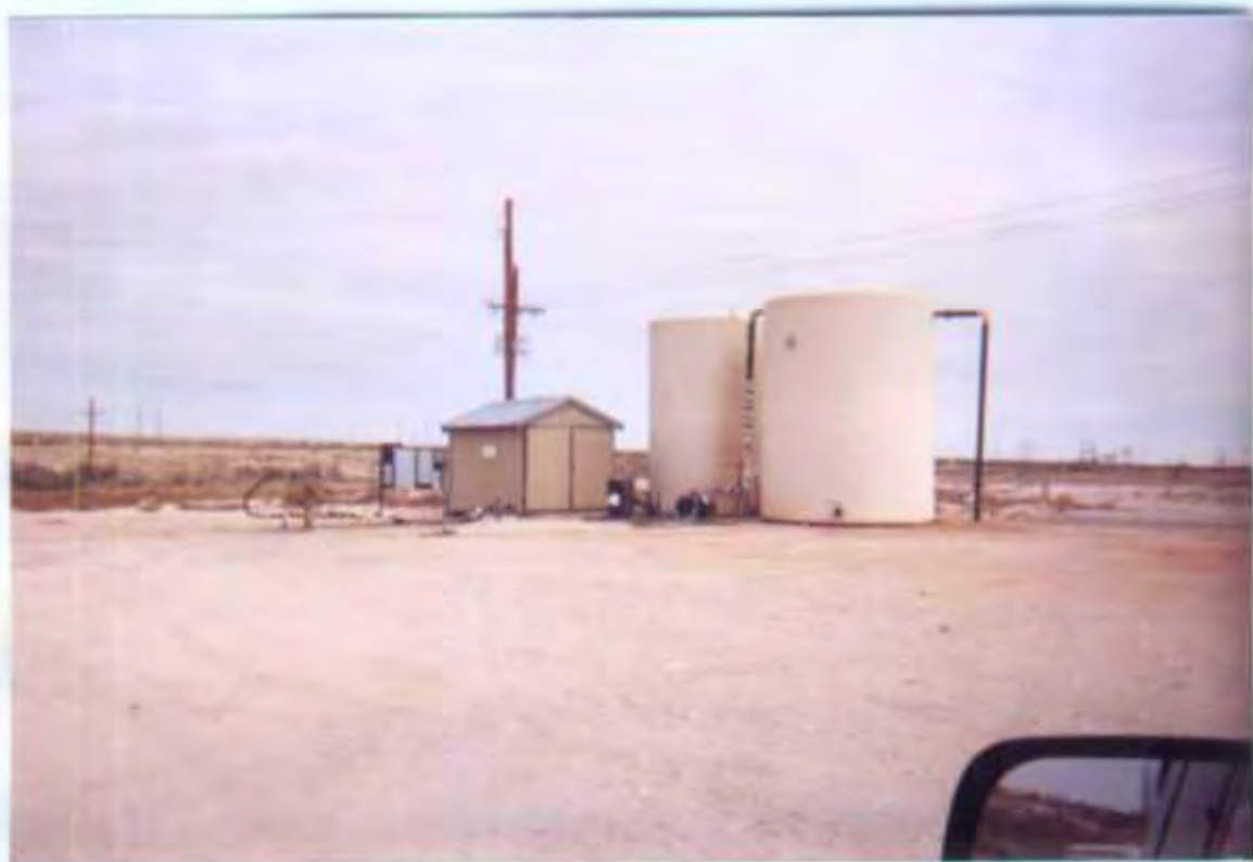
Brine Well, Pump house, Fresh water TANKS.
