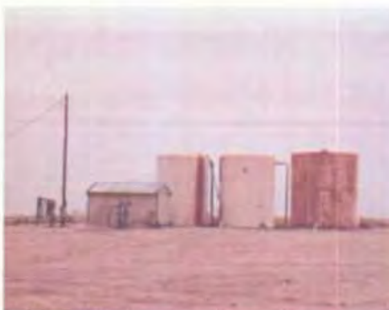
Fresh and Brine Water Tank Battery Unit
