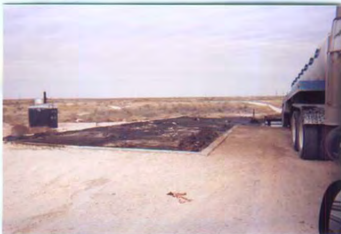
Cement Slab for Solids Out of Wash Pit
