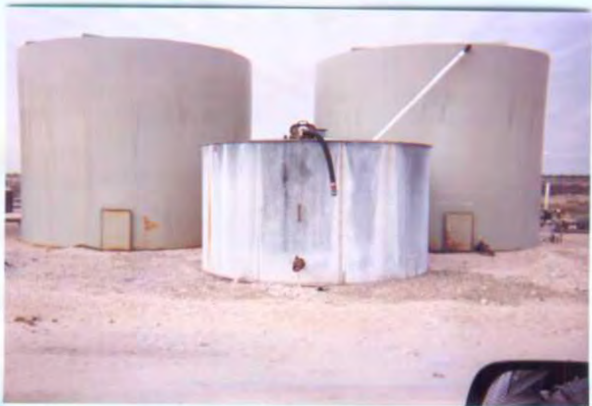
CATCH TANK for Brine Tanks
