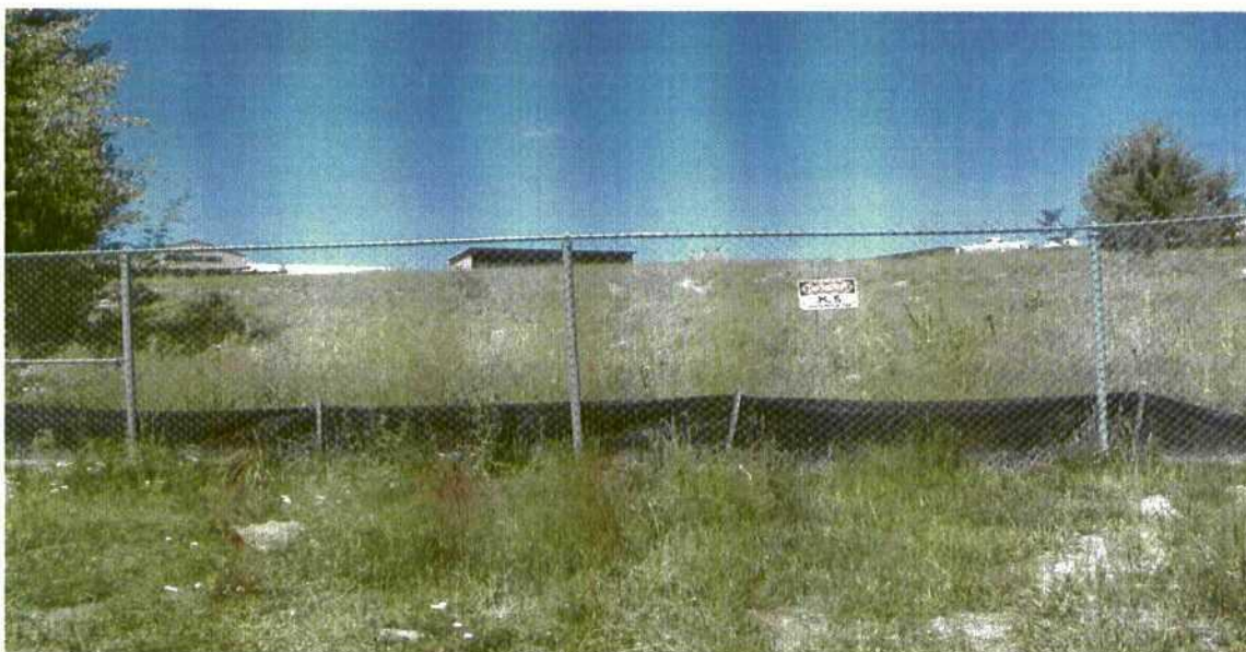
Looking Up Burns Swale at the HDR Perimeter Fence
