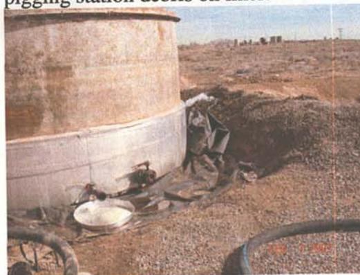
**Photo 6** – Near pigging station condensate container. Disrupted liner.
