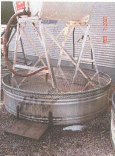
**Photo 8** – Lance service Co's product tanks with insufficient secondary containment.
